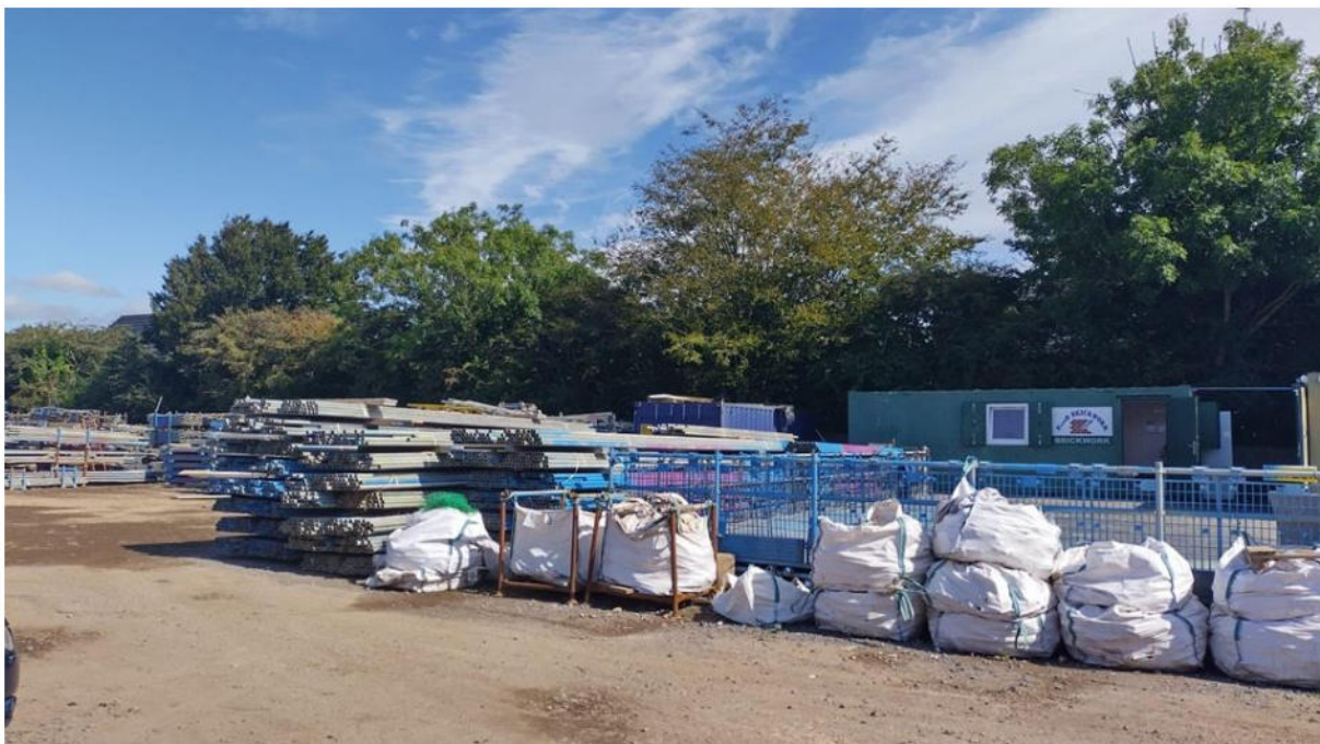
Figure 7: Site offices and storage area
