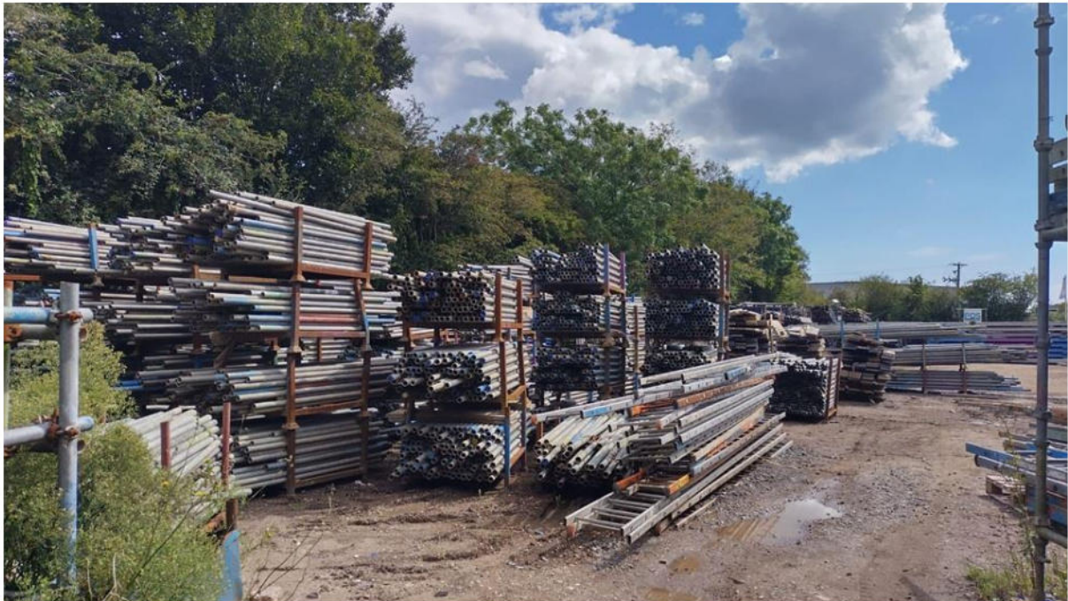
Figure 10: Storage of scaffold equipment
