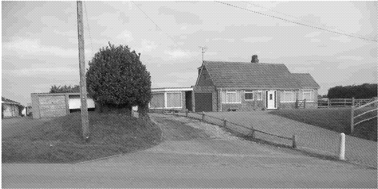
Figure 2: The Existing Site Access
