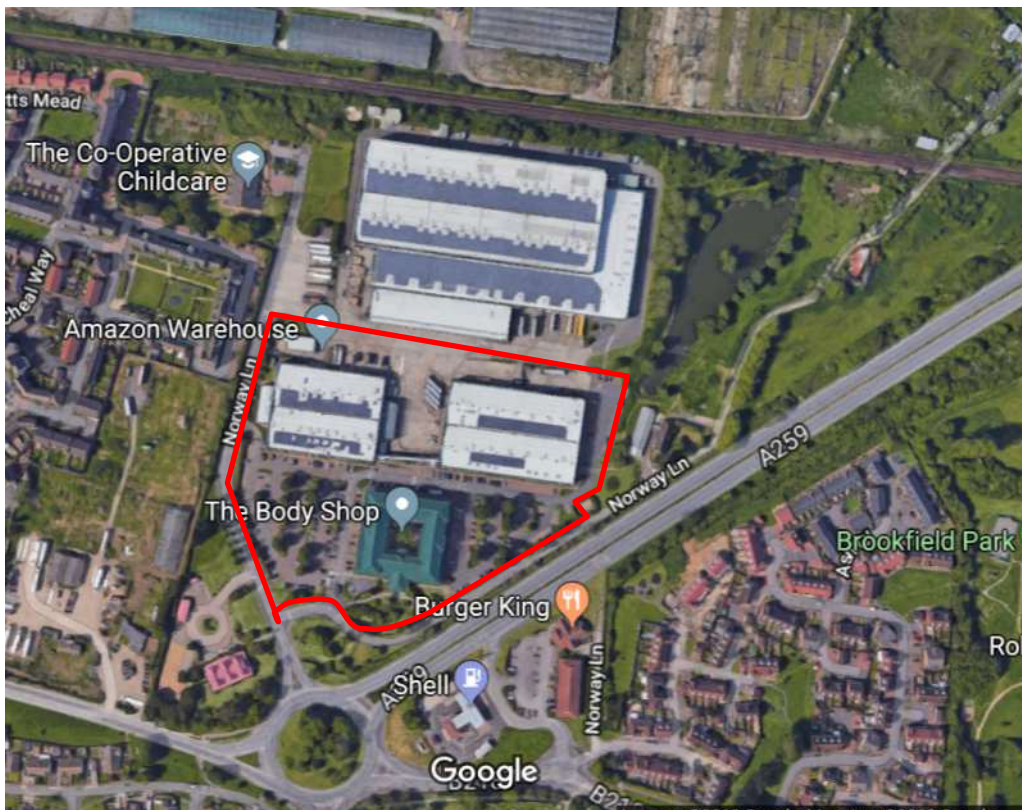
Figure 1.1 – Aerial View of the existing development site (approximate site boundary edged red)
