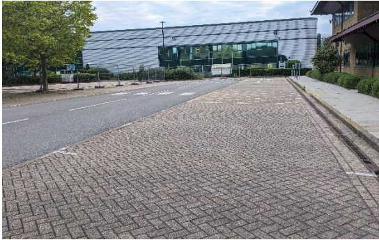
Photo 1: Hardstanding to the south of building B3.
