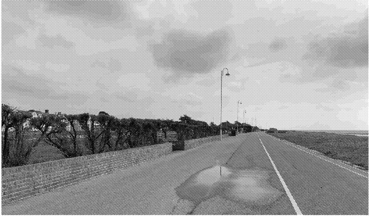
Fig 4. Photograph of Site E looking east
