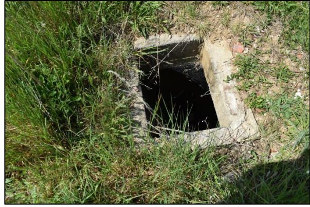
Plate 13: Opening to culvert/septic tank
