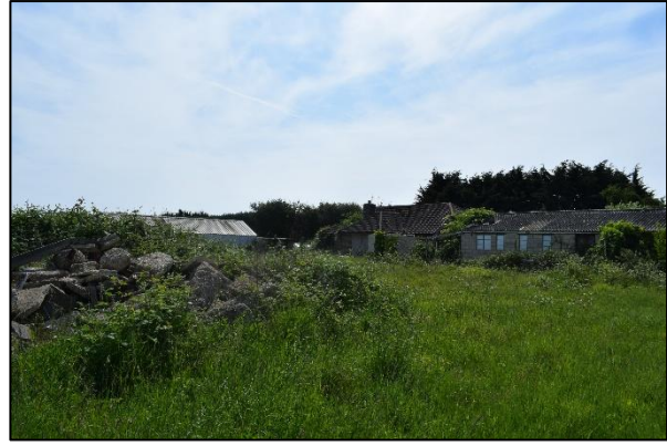
Plate 19: Concrete rubble in north of Site
