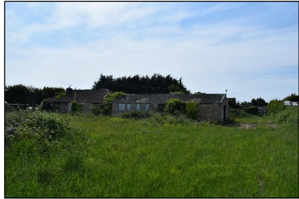
Plate 6: Dwelling and outbuildings looking south-east
