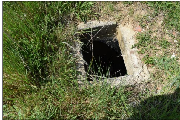
Plate 13: Opening to culvert/septic tank
