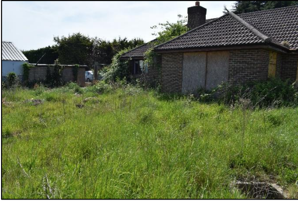
Plate 12: Location of culverts/septic tanks looking south-east
