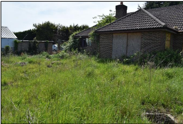
Plate 12: Location of culverts/septic tanks looking south-east
