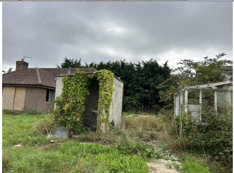
Photograph 12: Building 3. Ivy growth can be seen.
