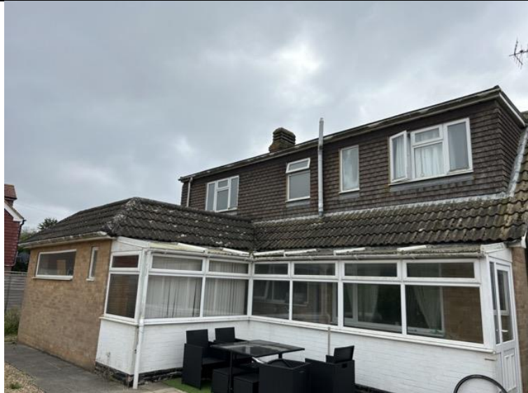
Photograph 4: Northern aspect of building 5.
