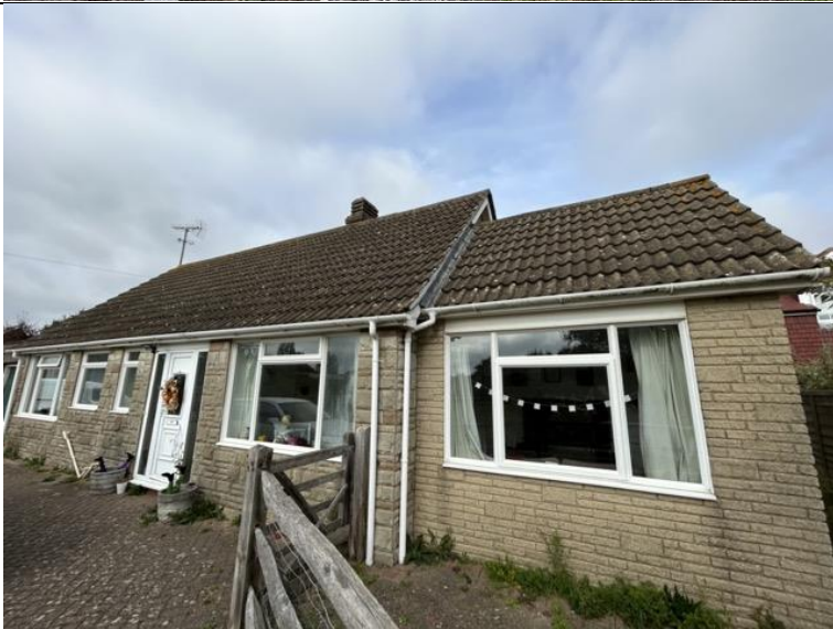
Photograph 6: Southern aspect of building 5.
