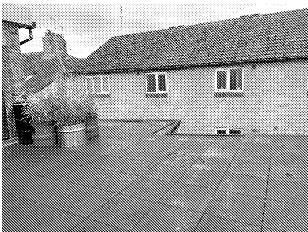
Photo 6: View west from application building toward Drummond Court
