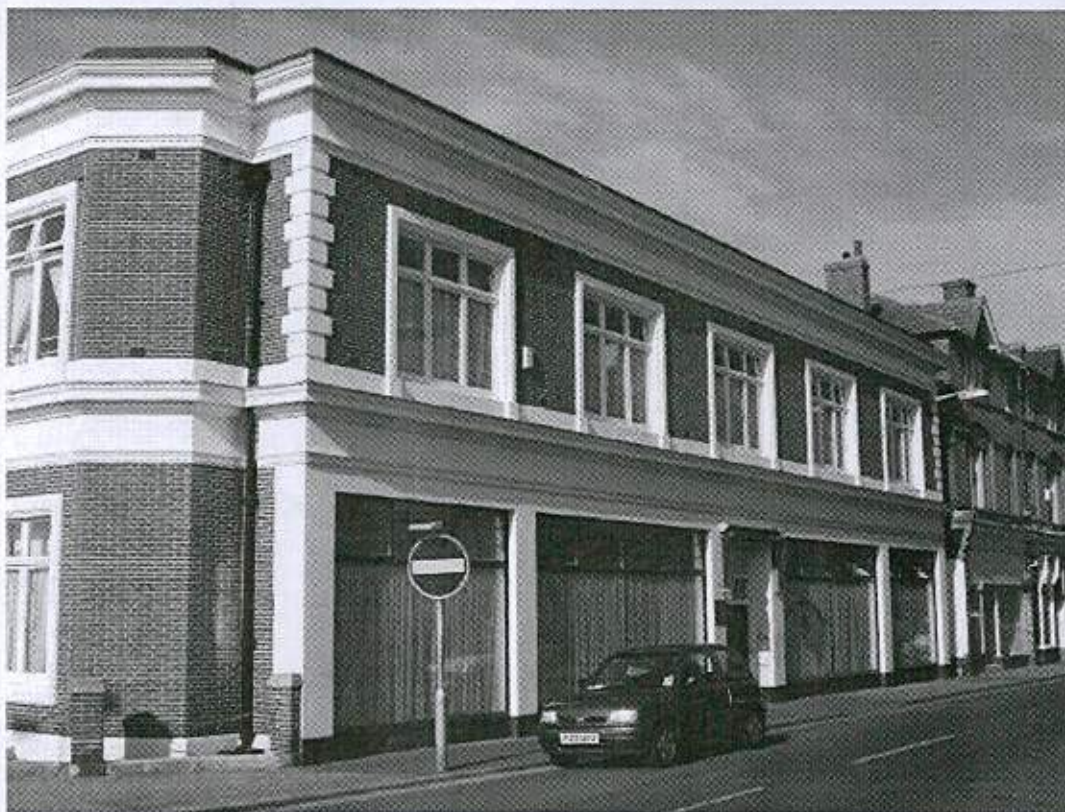
Photo 1 – East Elevation (Beach Road)
