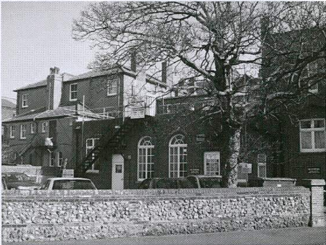
Photo 4 – Part view of West Elevation (New Road)
