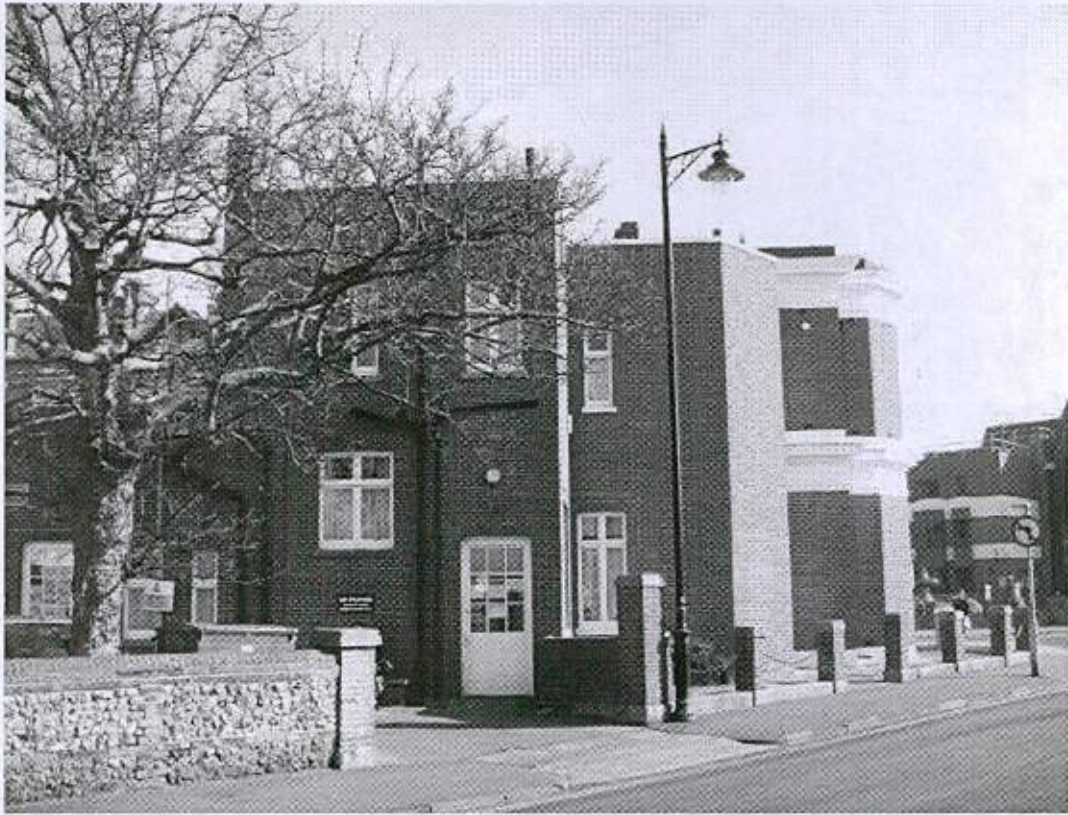
Photo 3 – Part view of West Elevation (New Road)
