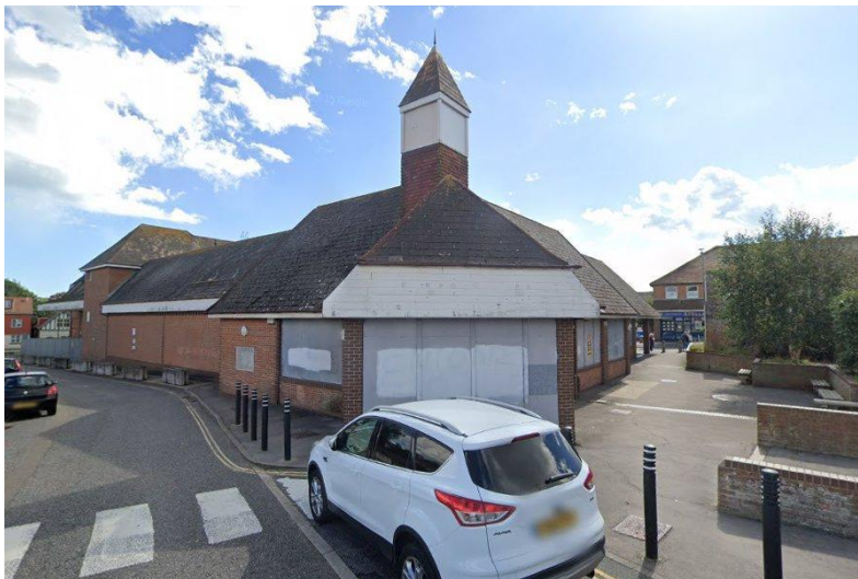
The former Waitrose site on Avon Road, Littlehampton (Image: Google Maps)
