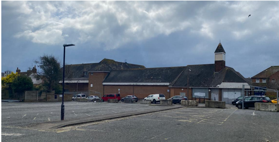
View south from the car park of the supermarket's north elevation
