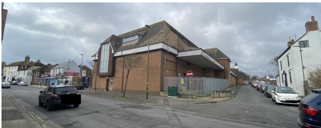
View west from East Street along Avon Road and of the supermarket's east and north elevations
