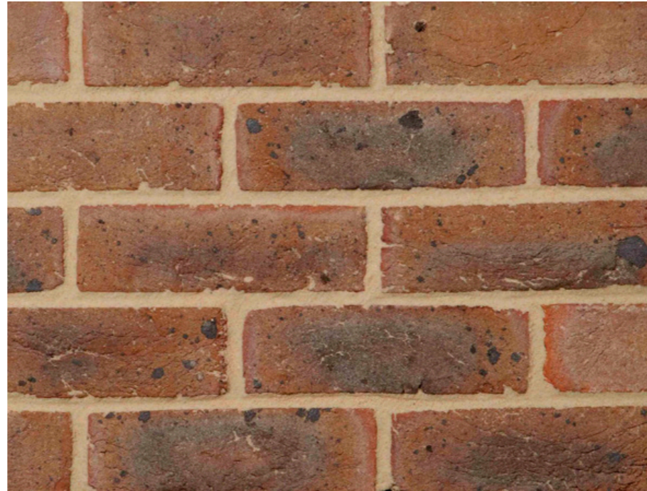
Red Brickwork to main elevations above plinth level.
