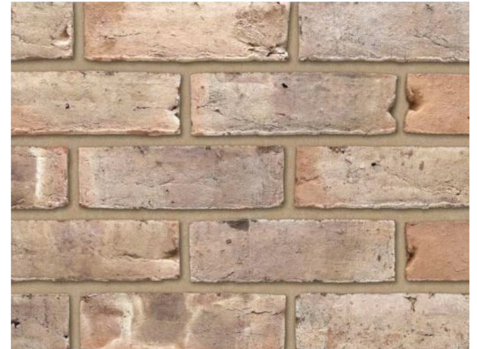
Buff Brickwork to main elevations above plinth level.
