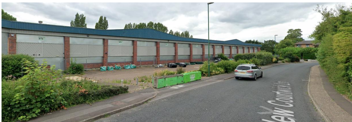
Figure 3 - Access to Site from South of New Courtwick Lane
