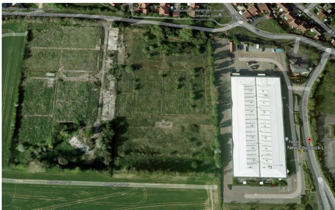
Figure 2 - Aerial Imagery of the Site
