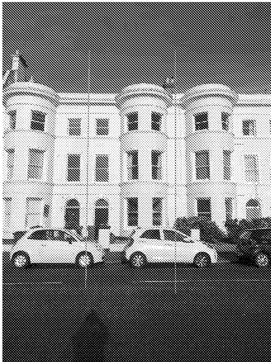
View of the front of the existing property.
