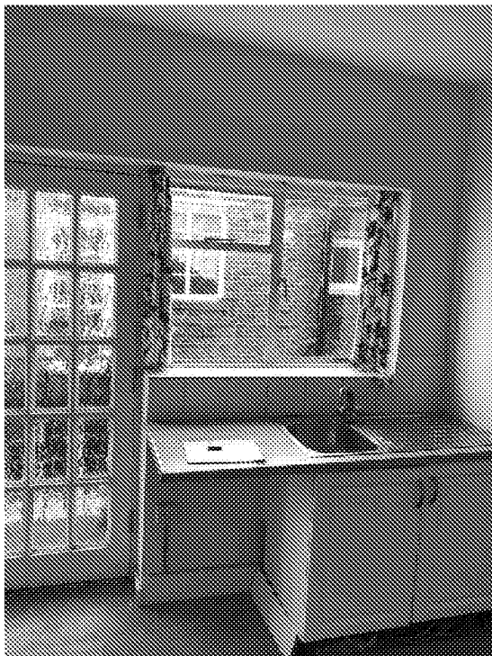
Existing glazed door and window to kitchen Proposed to be replaced.
