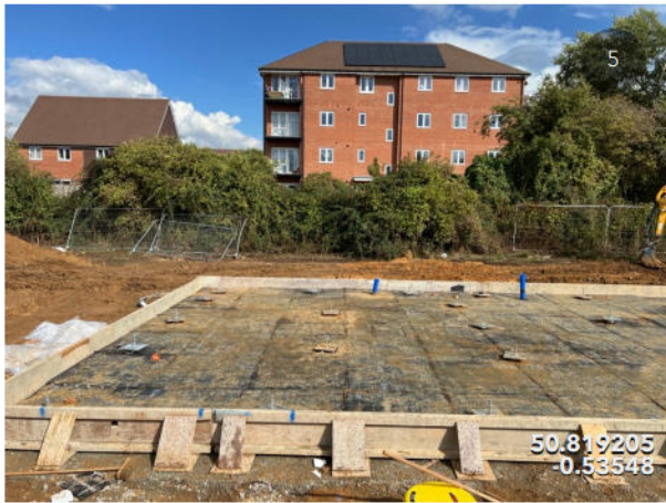
Rebar Works 1st layer and 2nd layer
