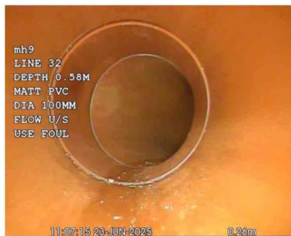
L32X_a653e029-9f5b-4e61-be3b-7592023faccd_20250701_1 70803_809.jpg, 00:00:08, 0.26 m Line deviates right
