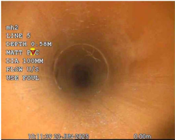
L5X_3042f87b-d10b-437e-858d-c84ca3e770ea_20250701_16 5720_869.jpg, 00:00:00, 0.00 m Start node, manhole, reference: FIC2
