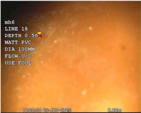
L18X_71753cfd-526d-4b79-986c-b3174321c1a7_20250701_170111_730.jpg, 00:00:00, 0.00 m Start node, manhole, reference: FIC5
