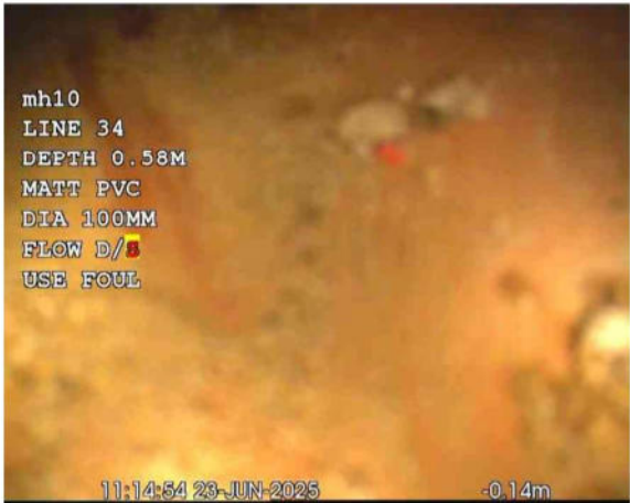
MH 10X_2cbfc18d-a6a1-41fa-a0d2-7c275e7a450a_20250701_17 0821_815.jpg, 00:00:00, 0.00 m Start node, manhole, reference: FIC9
