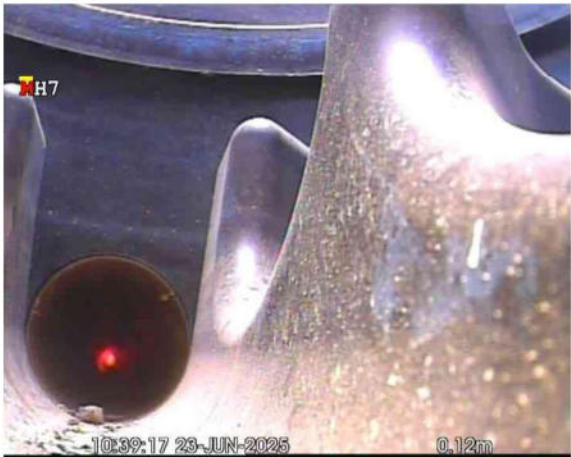
MH 7X_5941bba7-bcc6-4bff-b777-35939dffe072_20250701_1701 31_841.jpg, 00:00:07, 0.12 m Finish node, manhole, reference: FIC6
