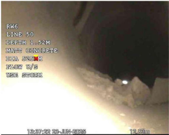
RW 6X_a3597531-0668-4c4c-8051-6e759ca75387_20250701_17 1256_231.jpg, 00:00:35, 12.83 m Connection other than junction at 9 o'clock, 150mm dia
