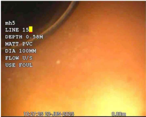
L15X_ee47413a-f90d-4052-9078-b98d4a60baaa_20250701_170004_497.jpg, 00:00:00, 0.00 m Start node, manhole, reference: FIC4
