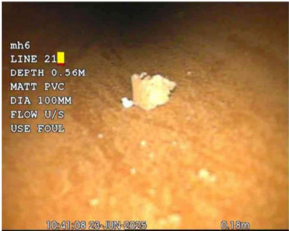
L21X_3362d6ac-9d56-4fcb-a30b-61576191f540_20250701_1 70148_977.jpg, 00:00:00, 0.00 m Start node, manhole, reference: FIC5
