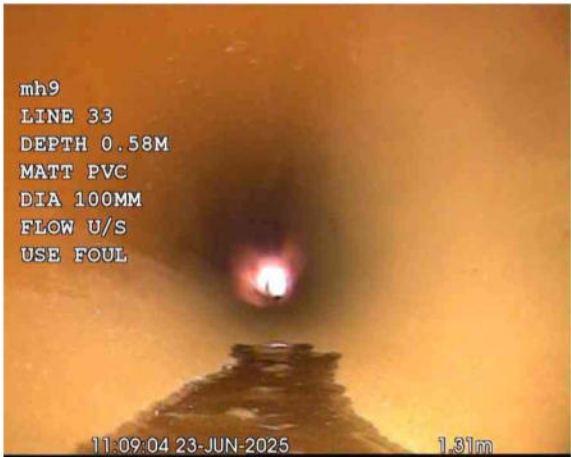
L33X_1e2cc001-e770-4413-b151-5020a8396adb_20250701_ 170814_568.jpg, 00:00:09, 1.31 m Water level, 5% of the vertical dimension
