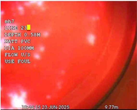
L23X_78767e09-2e67-400c-b39e-9a8d570b83f3_20250701_1 70224_543.jpg, 00:00:31, 9.77 m Finish node, other special chamber, reference: L23
