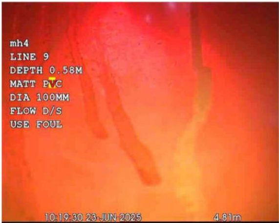
L9X_2ba4e900-a9a3-4dfc-9655-e23d937e7362_20250701_165859_796.jpg, 00:00:19, 4.81 m Finish node, other special chamber, reference: L9
