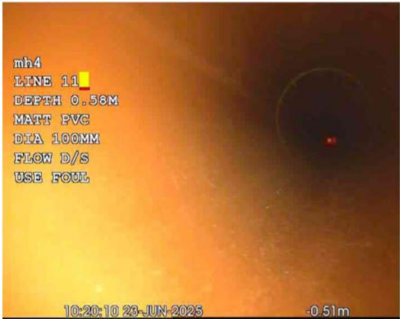
L11X_767c4a3c-b460-4a8c-b241-36e42d1a8127_20250701_165907_542.jpg, 00:00:00, 0.00 m Start node, manhole, reference: FIC3
