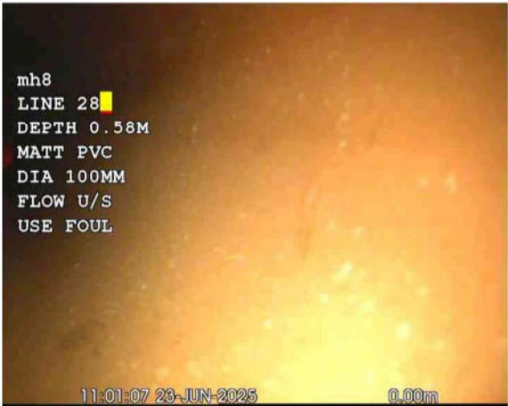
L28X_680eec6d-8221-4989-be09-cd10bb23a6d0_20250701_151458_645.jpg, 00:00:00, 0.00 m Start node, manhole, reference: FIC7
