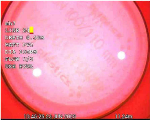
L24X_8cbdbb2f-8c2b-4f05-91ee-feded1350506_20250701_17 0244_398.jpg, 00:00:30, 11.24 m Finish node, other special chamber, reference: L24
