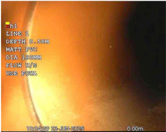
L1X_1bbf4d6f-35cd-4337-a4a3-12c395bffa7_20250701_165636_248.jpg, 00:00:00, 0.00 m Start node, manhole, reference: FIC1
