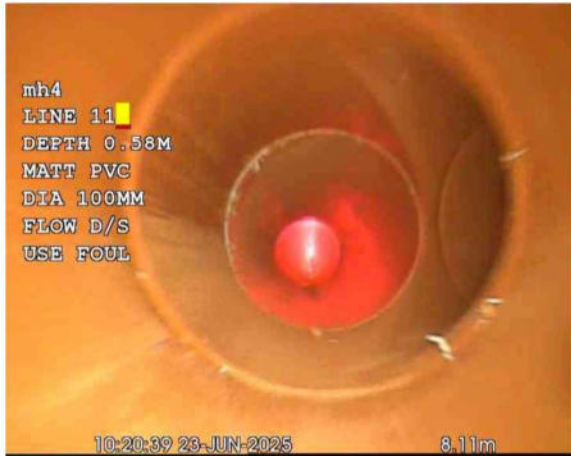
L11X_c108a6c0-ce4f-4e71-85a6-9047abcc196d_20250701_165908_983.jpg, 00:00:28, 8.00 m Junction at 3 o'clock, 100mm dia
