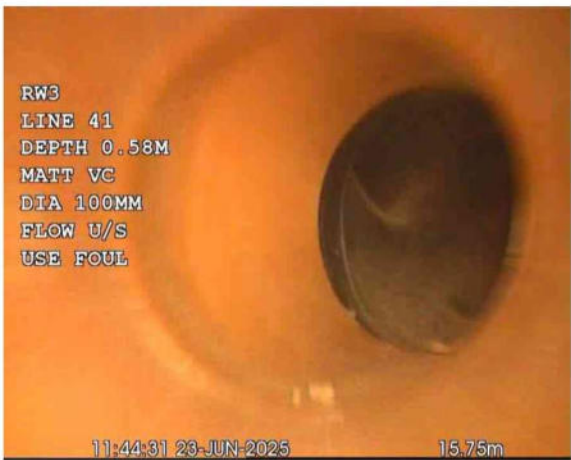
RW 4X_4a3d0c84-57e7-43e7-932e-ecde1b48e52d_20250701_17 1038_965.jpg, 00:00:46, 15.75 m Line deviates right
