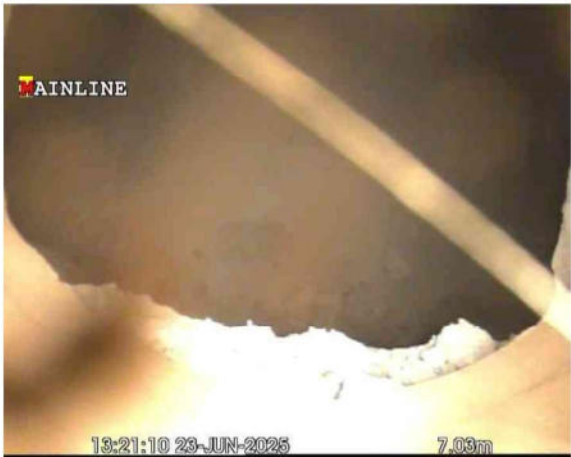
MH 17X_c161e9a8-ab15-4730-91e9-96ed611f1553_20250701_17 1202_241.jpg, 00:00:21, 7.03 m Finish node, major connection without manhole, reference: L47
