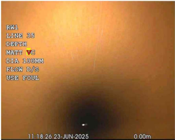
RW1X_17f319a1-05c0-444b-a076-ac21c78080f6_20250701_152835_305.jpg, 00:00:00, 0.00 m Start node, manhole, reference: PCPP1
