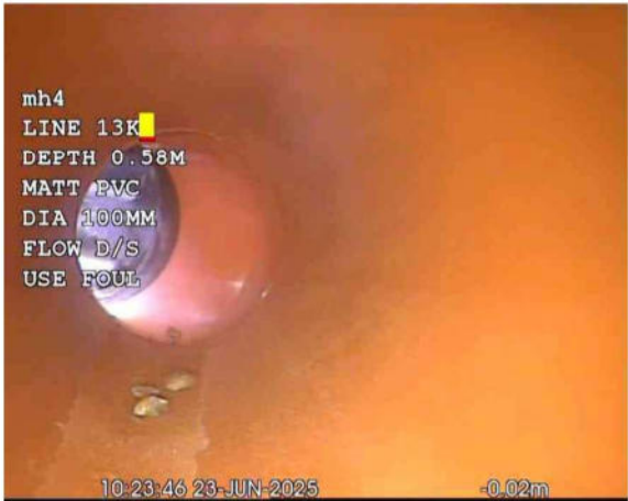
MH 4X_c86ac707-b44e-41be-9b42-eb888e8895f0_20250701_165 930_458.jpg, 00:00:00, 0.00 m Start node, manhole, reference: FIC3
