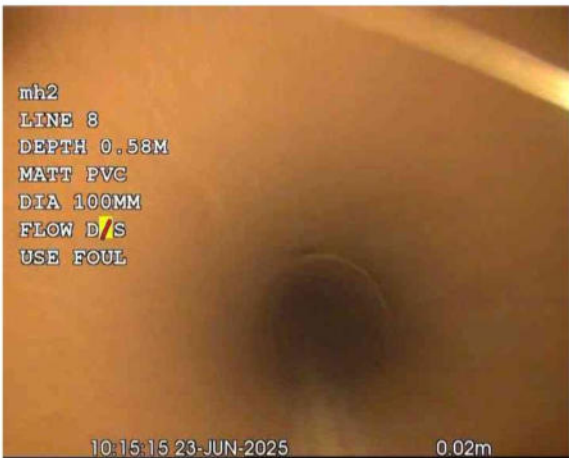
MH 2X_94e56988-60b4-400c-8ddf-b2c25e92e3cf_20250701_165820_496.jpg, 00:00:05, 0.02 m Pipe material changes to vitrified clay at this point
