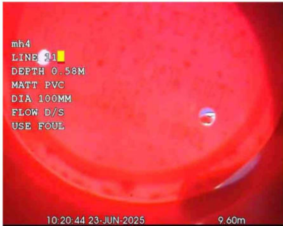
L11X_c727b411-ec56-4be1-96f4-f16a5e294fdc_20250701_165911_564.jpg, 00:00:33, 9.60 m Finish node, other special chamber, reference: L11
