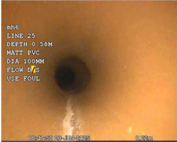
MH 6X_28a93d44-dc4d-4996-aa35-585673cb0242_20250701_17 0253_926.jpg, 00:00:08, 0.22 m Pipe material changes to vitrified clay at this point
