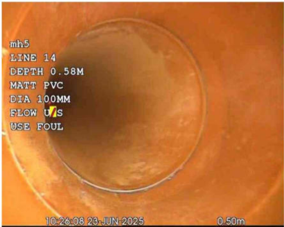
L14X_1b6d1808-0998-4c7c-8f52-ef9d7cade173_20250701_1 65943_387.jpg, 00:00:06, 0.59 m Line deviates left
