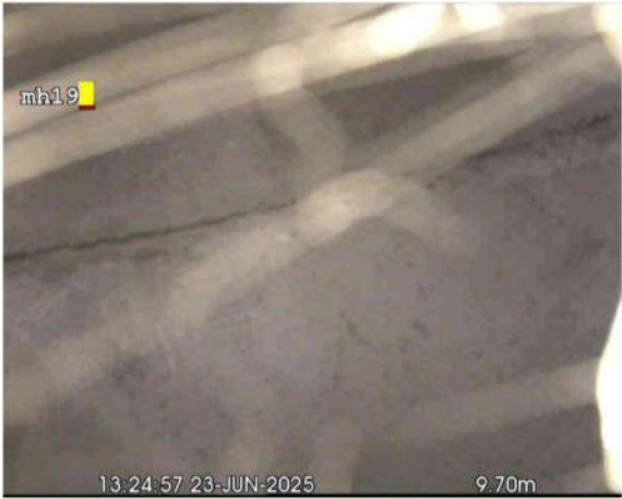
MH 18X_202dd446-6da3-4391-ad8d-15a0a9b2aed1_20250701_1 71213_817.jpg, 00:00:39, 9.70 m Finish node, manhole, reference: FMH78
