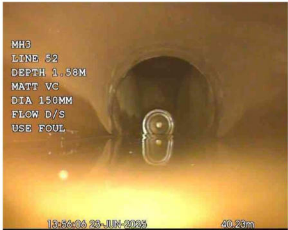
MH 3X_c2314810-71d2-42b8-a1a5-269413f999c8_20250701_171359_152.jpg, 00:01:28, 40.23 m Finish node, manhole, reference: FMH59
