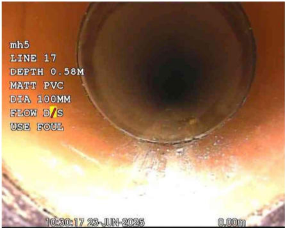
MH 5X_9c7c546a-2809-48f7-af21-f5dc52fd9237_20250701_1700 32_703.jpg, 00:00:00, 0.00 m Start node, manhole, reference: FIC4
