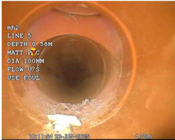
L5X_938a87fe-7f62-4631-9572-b758cfe81fa2_20250701_165 722_310.jpg, 00:00:15, 4.70 m Junction at 12 o'clock, 100mm dia
