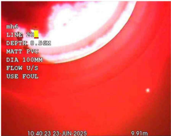
L20X_dbfad9c3-6daf-459a-aef1-d013eb22457f_20250701_17 0140_997.jpg, 00:00:27, 9.91 m Finish node, other special chamber, reference: L20
