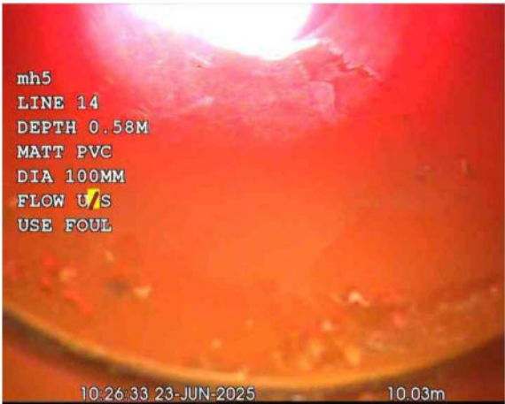
L14X_41cd12fc-dfbb-47c9-af25-f1598ffb512b_20250701_165947_739.jpg, 00:00:31, 10.03 m Finish node, other special chamber, reference: L14
