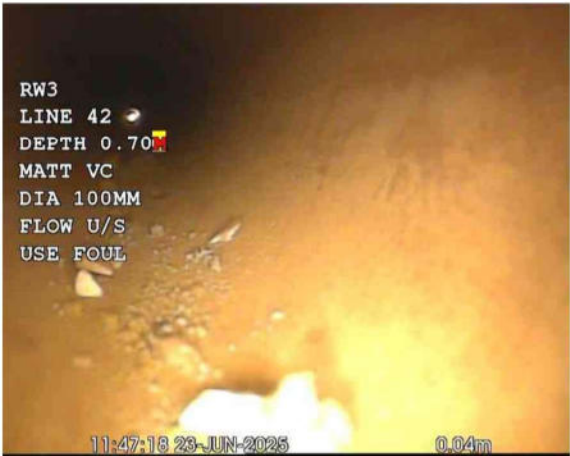
L42X_b19ed3d1-e8ac-49b8-bcbc-5ecef1a1e853_20250701_171102_905.jpg, 00:00:00, 0.00 m Start node, manhole, reference: SMH49
