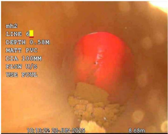
L6X_325c04bb-f860-406e-8a77-e51080b36ace_20250701_16 5740_681.jpg, 00:00:28, 8.68 m Line deviates up
