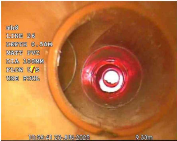
L26X_2d7e3045-ccc4-4a4c-9202-c453bad45397_20250701_170332_782.jpg, 00:00:33, 9.33 m Junction at 9 o'clock, 100mm dia
