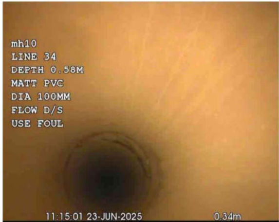
MH 10X_d9c31105-c8fa-4a63-8956-95dd5c9a69ad_20250701_17 0822_692.jpg, 00:00:07, 0.34 m Pipe material changes to vitrified clay at this point
