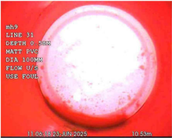
L31X_18350002-44d5-4eaf-80ba-452eaa3bf113_20250701_1 70756_338.jpg, 00:00:36, 10.53 m Finish node, other special chamber, reference: L31
