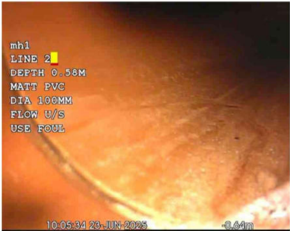
L2X_2511c4da-2cc1-462c-a3ae-c4b7dc92e414_20250701_16 5650_134.jpg, 00:00:00, 0.00 m Start node, manhole, reference: FIC1
