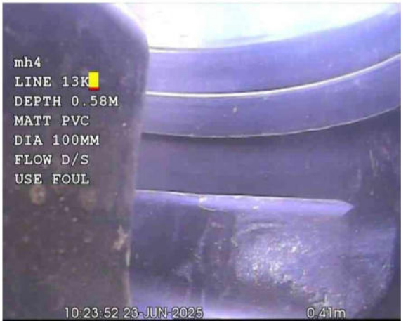
MH 4X_41e1036d-36e2-4be6-8a46-be6c787ce542_20250701_16 5932_631.jpg, 00:00:07, 0.41 m Finish node, manhole, reference: FIC4
