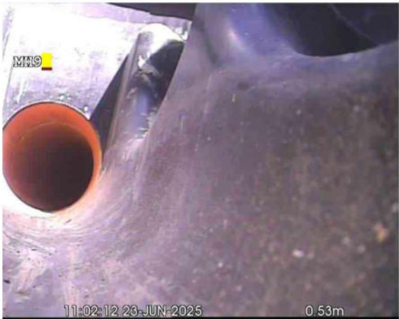
MH 9X_9f2d9121-05dc-4e93-8318-28fba525ce9e_20250701_170 723_381.jpg, 00:00:08, 0.53 m Finish node, manhole, reference: MH 9
