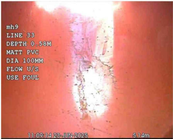
L33X_45c437ca-615a-4fc3-b1de-97e3714f5d1f_20250701_17 0815_782.jpg, 00:00:19, 5.14 m Line deviates up
