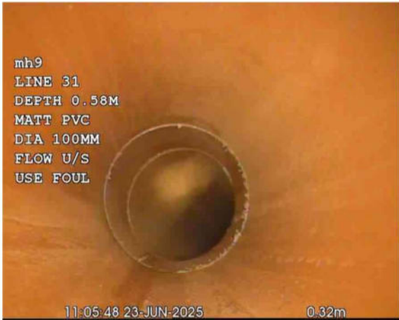
L31X_3b2e0d3d-8fa8-4fc7-a71a-8be422023423_20250701_170752_924.jpg, 00:00:06, 0.32 m Line deviates right
