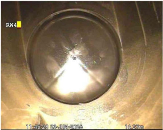
RW 4X_4293e051-128e-43bd-af61-42012154903d_20250701_17 1040_244.jpg, 00:00:52, 16.27 m Finish node, manhole, reference: PPCP2
