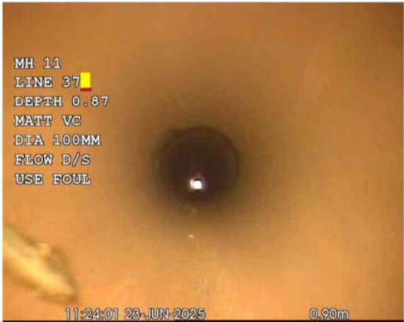
MH 11X_f9c60126-d79b-426f-ad26-8be088aa6ce7_20250701_17 0907_112.jpg, 00:00:06, 0.90 m Pipe material changes to vitrified clay at this point
