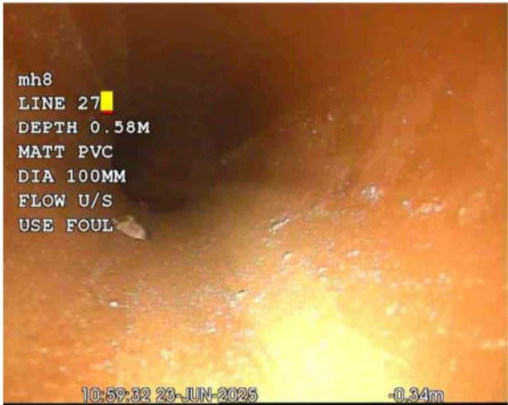
L27X_6e79de81-231d-41d5-8f39-2fcb37537f0b_20250701_170656_245.jpg, 00:00:00, 0.00 m Start node, manhole, reference: FIC7
