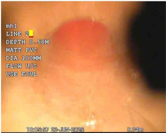
L2X_58c295d6-6d6b-47d4-baf9-7f201caeab20_20250701_16 5653_361.jpg, 00:00:23, 8.94 m Line deviates up
