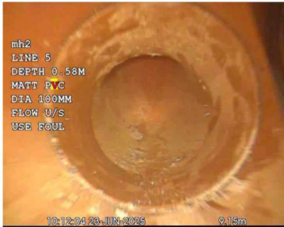
L5X_6477f5c9-64de-4ead-b229-b5a59f14c18e_20250701_16 5725_068.jpg, 00:00:26, 9.15 m Line deviates up
