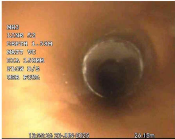
MH 3X_f1f45171-fd3f-45b6-89f7-ecc838128f44_20250701_171355_430.jpg, 00:00:48, 26.15 m Junction at 3 o'clock, 100mm dia
