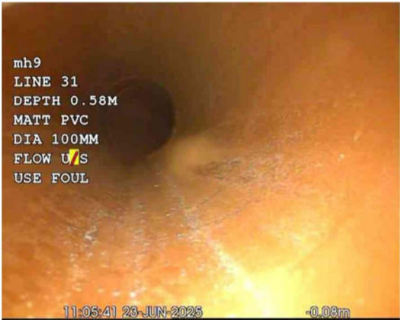
L31X_7b19a8f0-dca6-4bb9-b6b3-050d38c26002_20250701_170752_079.jpg, 00:00:00, 0.00 m Start node, manhole, reference: FIC8
