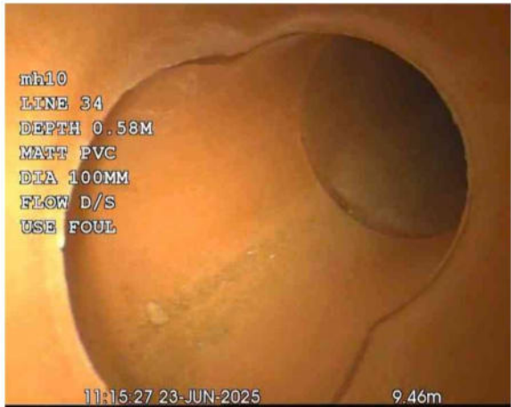
MH 10X_adbcc411-c696-410b-b1b7-faa9e9a4c3ce_20250701_17 0825_407.jpg, 00:00:33, 9.46 m Finish node, major connection without manhole, reference: L34
