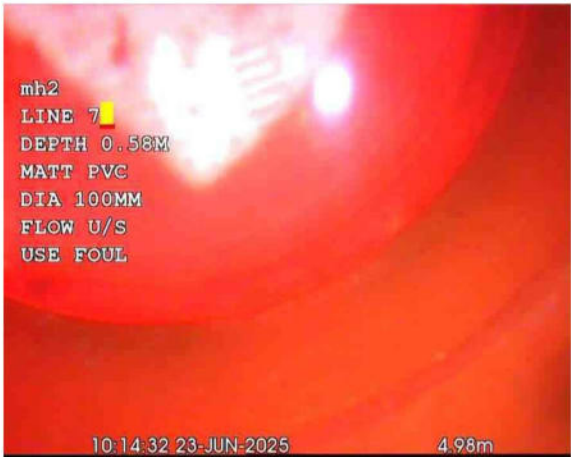
L7X_e935c35a-27c0-40c5-8911-1b3ede397993_20250701_1 65809_912.jpg, 00:00:24, 4.98 m Finish node, other special chamber, reference: L7
