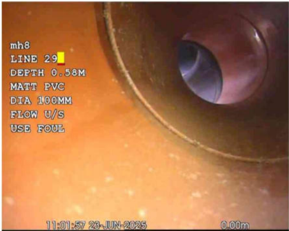
MH 9X_88411c36-58cb-4942-81a3-9a13ce137e3b_20250701_15 1617_761.jpg, 00:00:00, 0.00 m Start node, manhole, reference: FIC7
