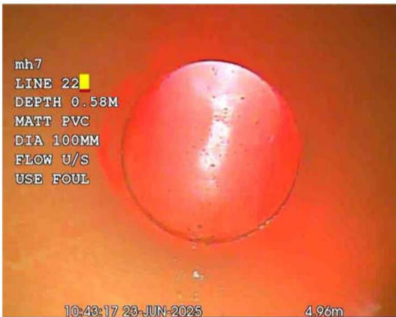
L22X_45675bc0-01f7-4c64-a830-67f27a4f2d40_20250701_170204_018.jpg, 00:00:16, 4.96 m Line deviates up
