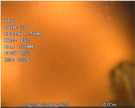
MH 8X_2bb9b6d8-11a1-4e71-9cf7-ddcdb8cee365_20250701_151 726_921.jpg, 00:00:00, 0.00 m Start node, manhole, reference: FIC7
