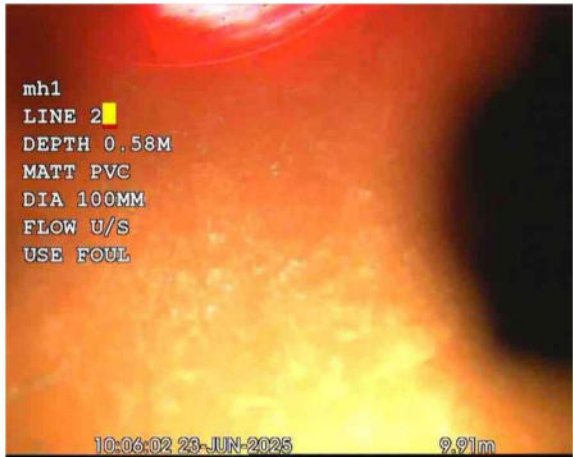
L2X_8929a665-5a73-4a0c-a776-ac0ec8cfeb3f_20250701_16 5654_537.jpg, 00:00:28, 9.91 m Finish node, other special chamber, reference: L2
