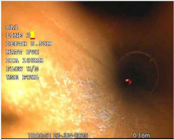
L3X_e10ebae3-6c2e-48ef-8aab-ca1c8fe4c35e_20250701_165659_651.jpg, 00:00:00, 0.00 m Start node, manhole, reference: FIC1
