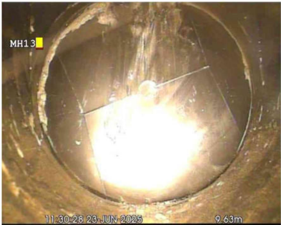
MH 13X_73656d1d-e237-4282-a5ae-75aa3a4f0259_20250701_170929_326.jpg, 00:00:28, 9.63 m Finish node, manhole, reference: FIC11
