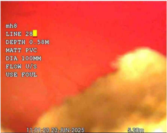
L28X_1db90be5-4416-4f6f-b51e-56d82223305d_20250701_170707_472.jpg, 00:00:17, 5.20 m Finish node, other special chamber, reference: L28
