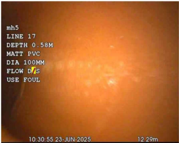
MH 5X_152f6aef-c0a4-48cc-a997-b37a8dd35f18_20250701_1700 37_506.jpg, 00:00:39, 12.29 m Finish node, major connection without manhole, reference: L17
