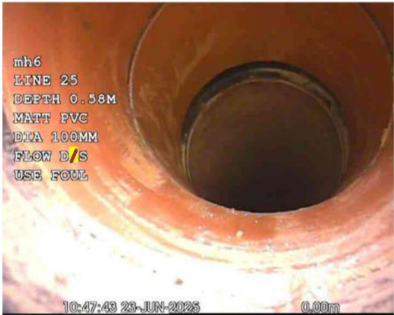
MH 6X_c6c58a00-b959-4740-9062-1bb79d81512e_20250701_15 0620_114.jpg, 00:00:00, 0.00 m Start node, manhole, reference: FIC5
