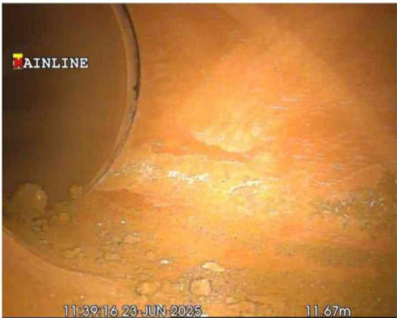
MH 15X_70693e50-5f42-4988-8b93-f4438a912902_20250701_171001_299.jpg, 00:00:31, 11.67 m Finish node, major connection without manhole, reference: L40
