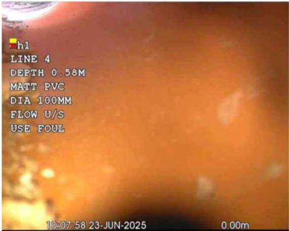
MH 1X_7628e776-9933-4dfa-9d46-dc22df8876ef_20250701_1657 14_434.jpg, 00:00:00, 0.00 m Start node, manhole, reference: FIC1
