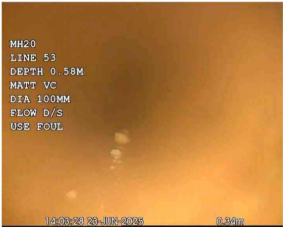
MH 20X_1a579186-68b0-4579-979a-5bfcdb216fde_20250701_17 1405_246.jpg, 00:00:04, 0.34 m Pipe material changes to vitrified clay at this point
