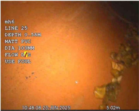
MH 6X_4c66a576-178d-44dd-8418-f414a370aa04_20250701_170 300_909.jpg, 00:00:26, 5.02 m Finish node, major connection without manhole, reference: L25
