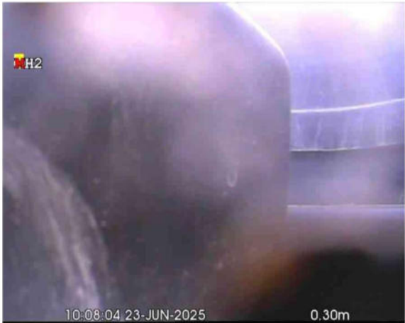
MH 1X_514b3128-7805-4a17-9427-a0a140d41911_20250701_16 5715_665.jpg, 00:00:07, 0.30 m Finish node, manhole, reference: FIC2
