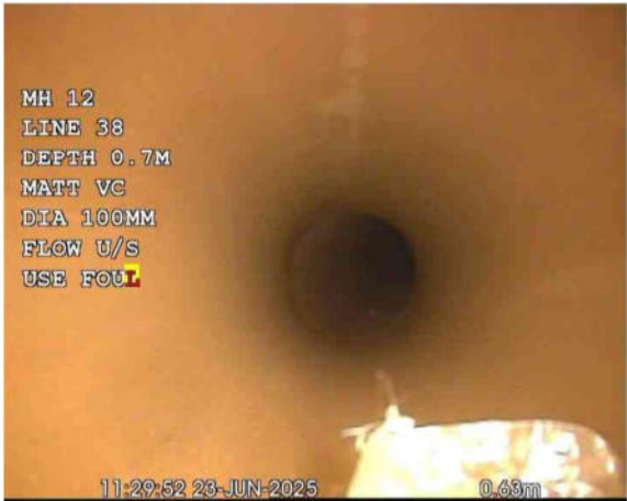
MH 13X_542487ce-bc2b-41e8-a440-7d6d188d7837_20250701_170926_996.jpg, 00:00:00, 0.00 m Start node, manhole, reference: FMH77
