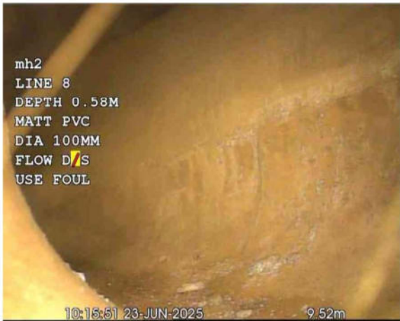
MH 2X_c00d62d1-8d8b-4452-b6e0-ec6d661688c0_20250701_16 5827_768.jpg, 00:00:41, 9.52 m Finish node, manhole, reference: FMH52
