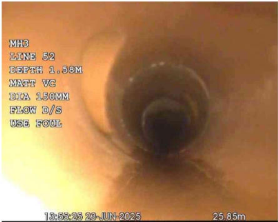
MH 3X_48989a1c-9e95-4c8e-8925-695b3b9f80b9_20250701_171354_153.jpg, 00:00:47, 25.85 m Junction at 9 o'clock, 100mm dia
