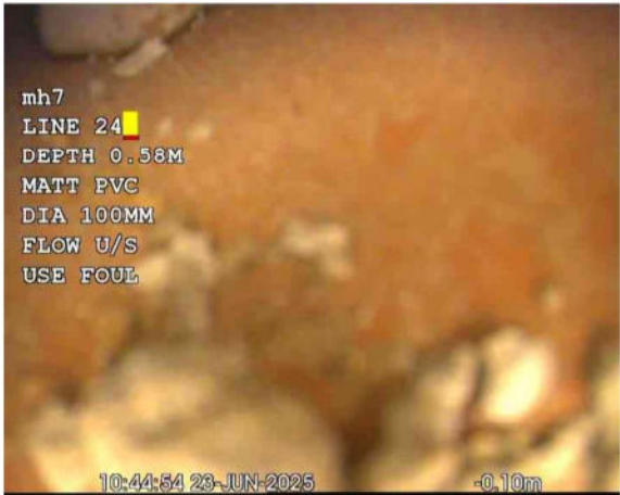
L24X_b3aecc8a-89fc-441c-9322-54aeb5668802_20250701_170239_547.jpg, 00:00:00, 0.00 m Start node, manhole, reference: FIC6
