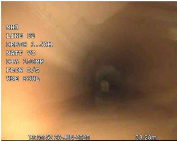
MH 3X_b00ace25-f294-404c-9763-72f83220d81c_20250701_171357_040.jpg, 00:01:14, 38.28 m Water level, 20% of the vertical dimension
