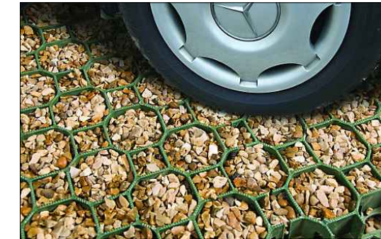
Example of Cellular Plastic Porous Paving System
