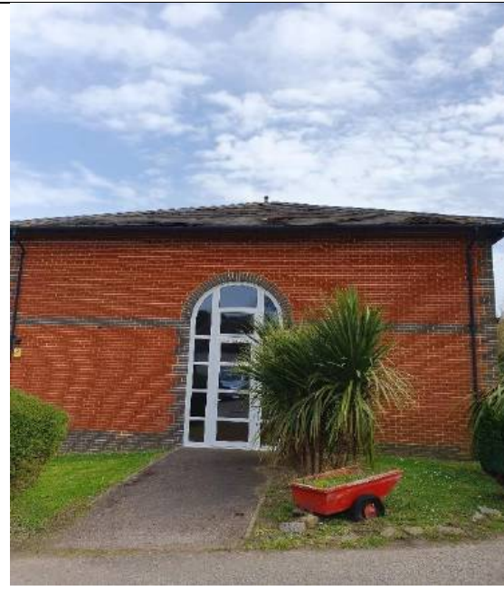
Photograph 6: External western elevation of B1.
