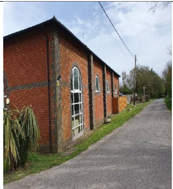
Photograph 8: External southern elevation of B1 with amenity grassland and introduced shrub.
