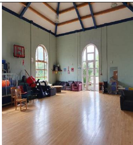
Photograph 4: Internal area of B1.
