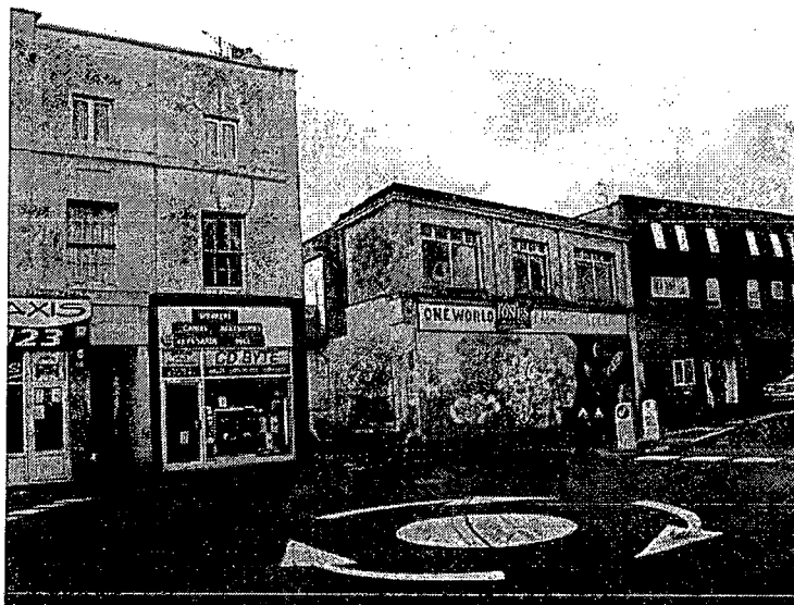
Terminus Road site access with existing boarded up former market building adjacent to the access.
