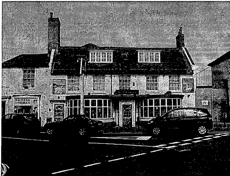
The Cob and Pen Public House Listed Structure
