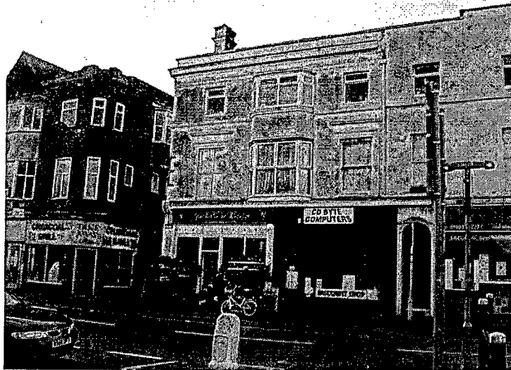
High Street access between existing retail units
