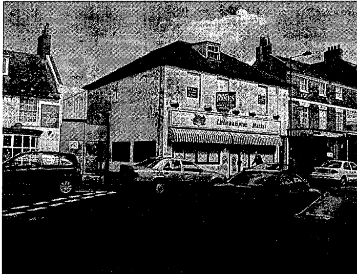
Surrey Street site access and existing retail unit with residential accommodation above.
