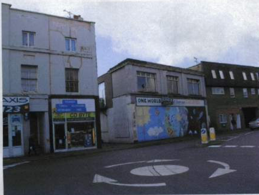
Terminus Road site access with existing boarded up former market building adjacent to the access.
