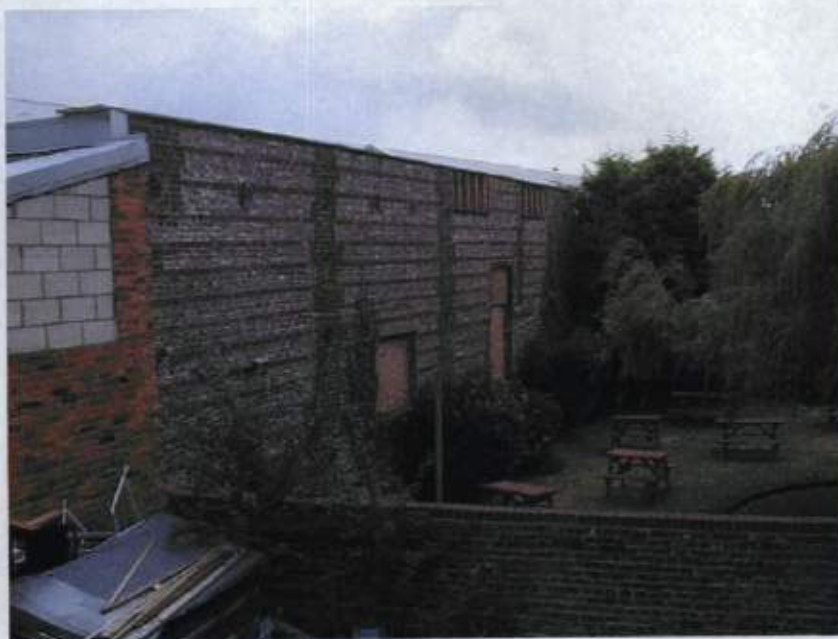
Boundary wall to Cob and Pen garden
