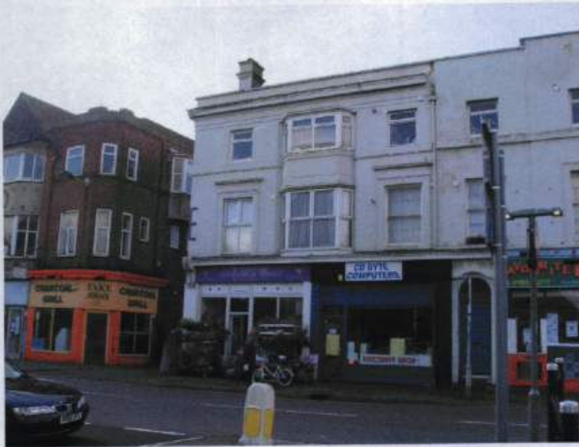
High Street access between existing retail units
