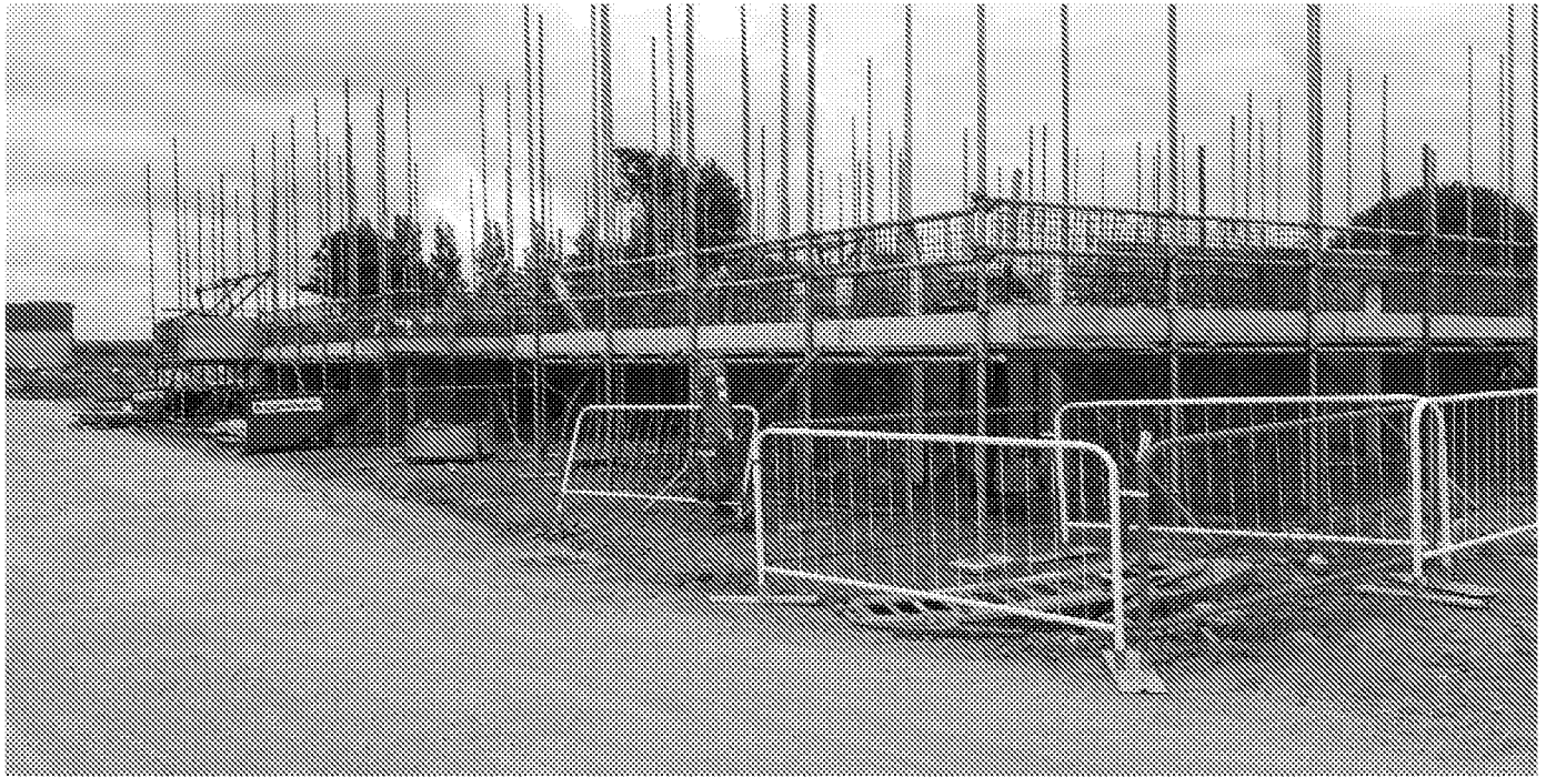
Plate 13 16th August 2019 - General Site - Plots 1 to 8 being built.
