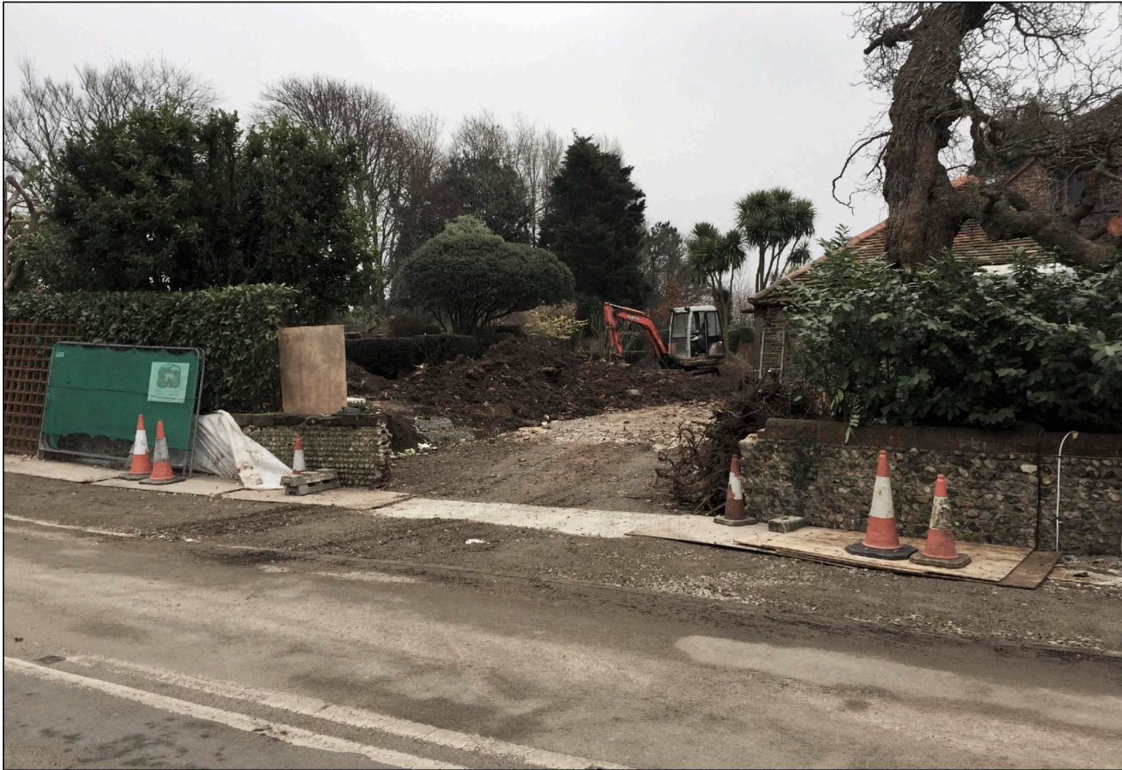
EXISTING SIDE ENTRANCE PHOTOGRAPH
