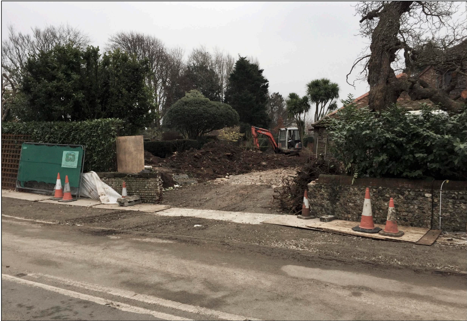
EXISTING SIDE ENTRANCE PHOTOGRAPH
