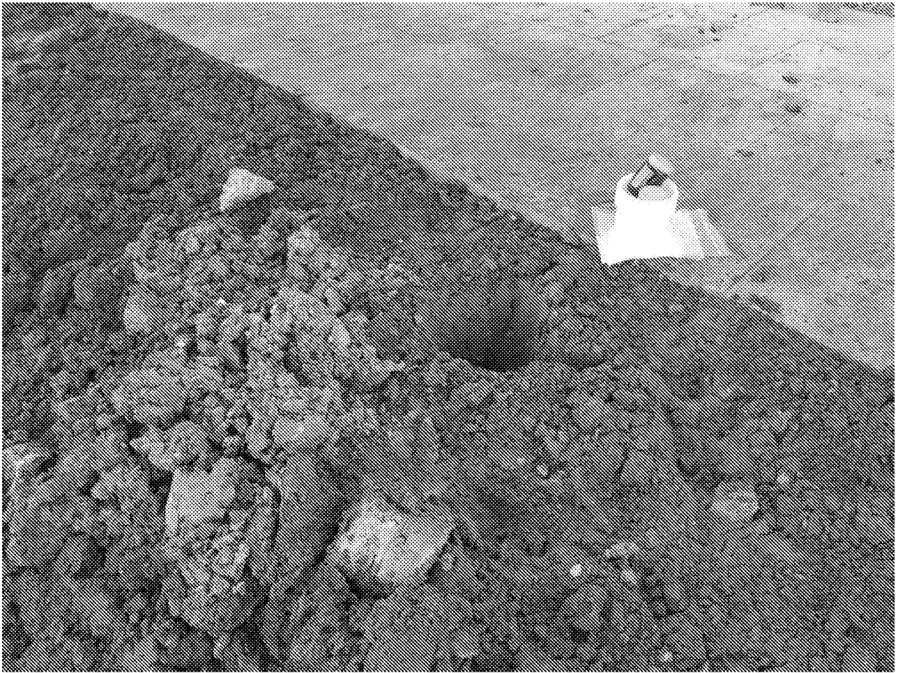
Photo of hole with tape in place
