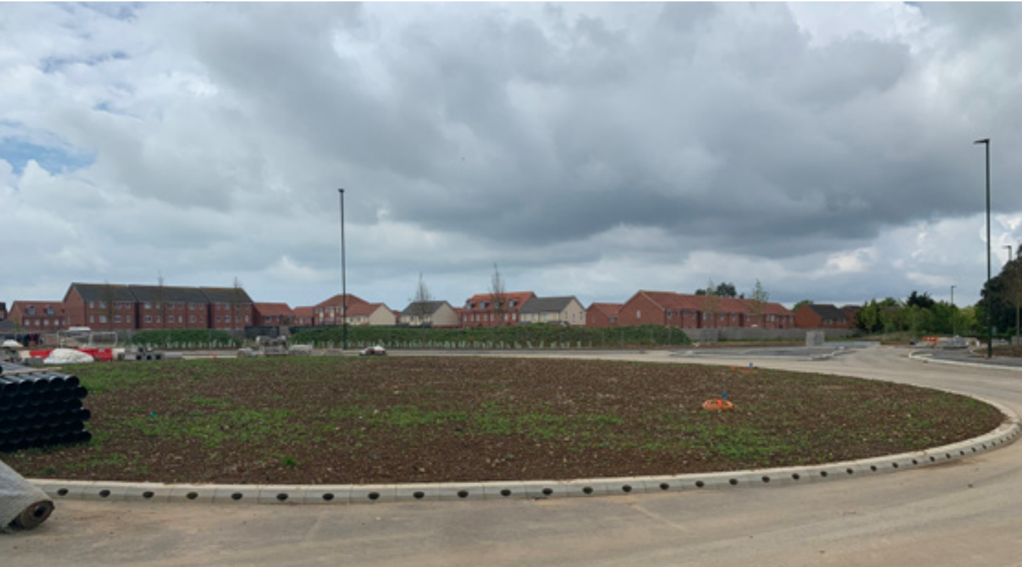
Fig. 10 - View 1 - View of New Roundabout from the Lyminster-Bypass
