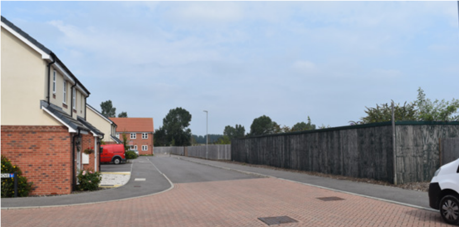
Fig. 12 - View 3 - View North showing Site A boundary condition on Hinchliff Drive
