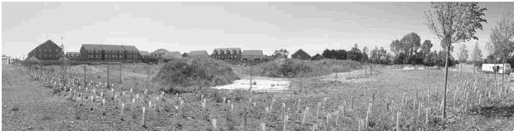
Photograph C - Lines of standard stock trees and hedgerow whips have been planted to the roadside edges to the boundaries of sites A and B.
