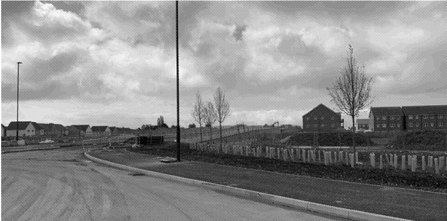
Fig. 13 - View 4 - View South along the Lyminster-Bypass
