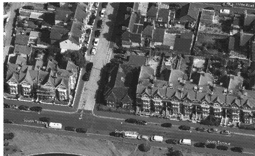
Aerial photo of surrounding site [Bing Maps]
