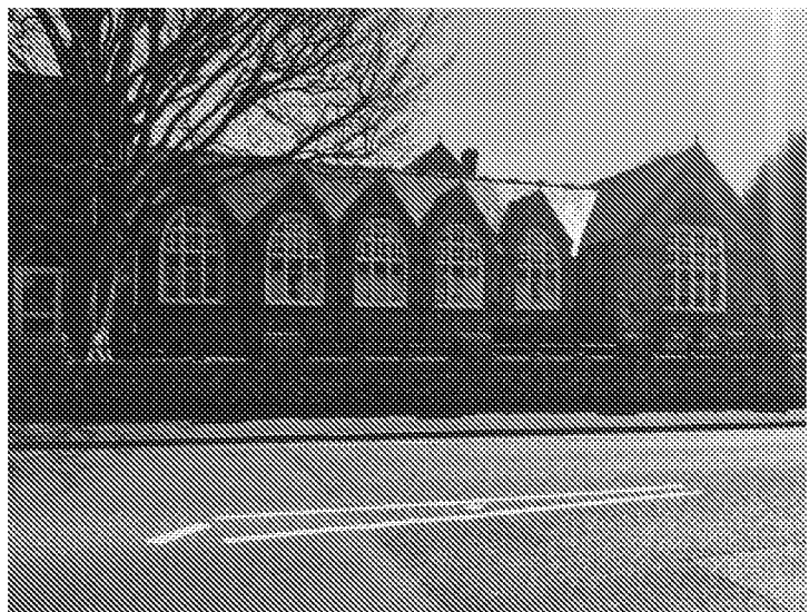
Figure 3.3 – East Street School (Youth Centre) and The Low Wall
