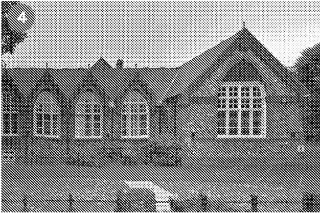
Flintstone Centre. Pitched roof
