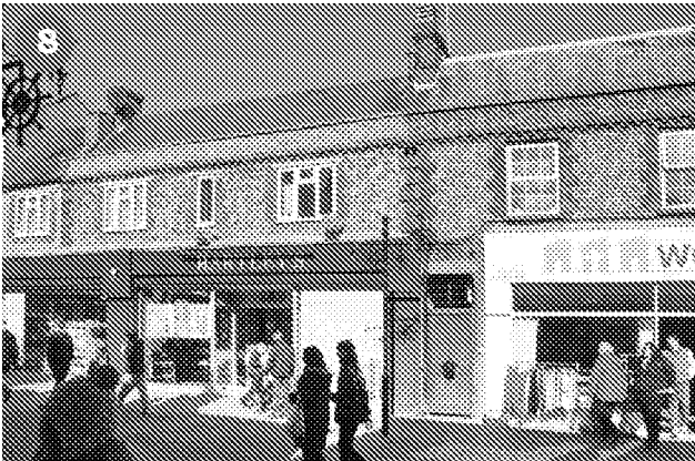
High Street, Pitched roof
