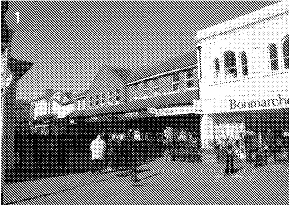
High Street. Mixed roof types
