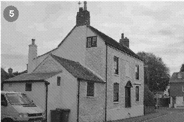
Avon Road. Pitched roof
