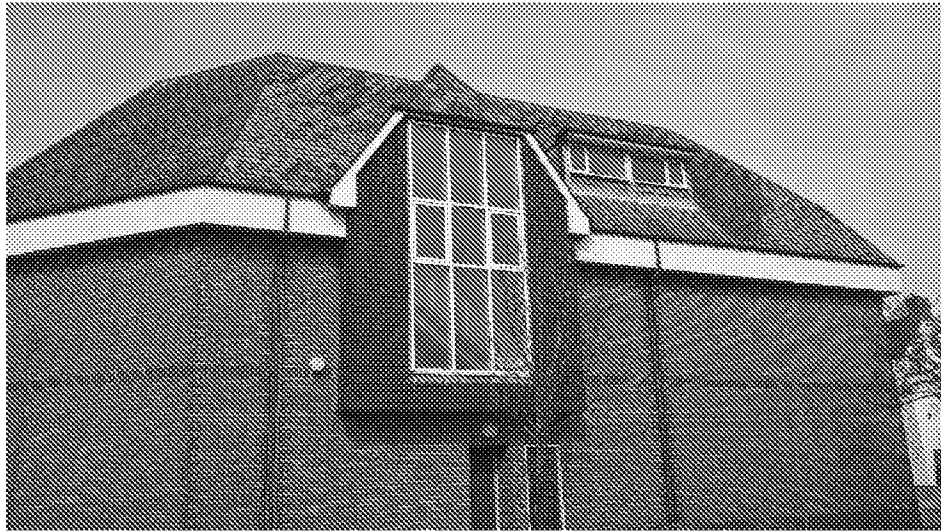
Plate 3 – View of the eastern elevation of B1.
