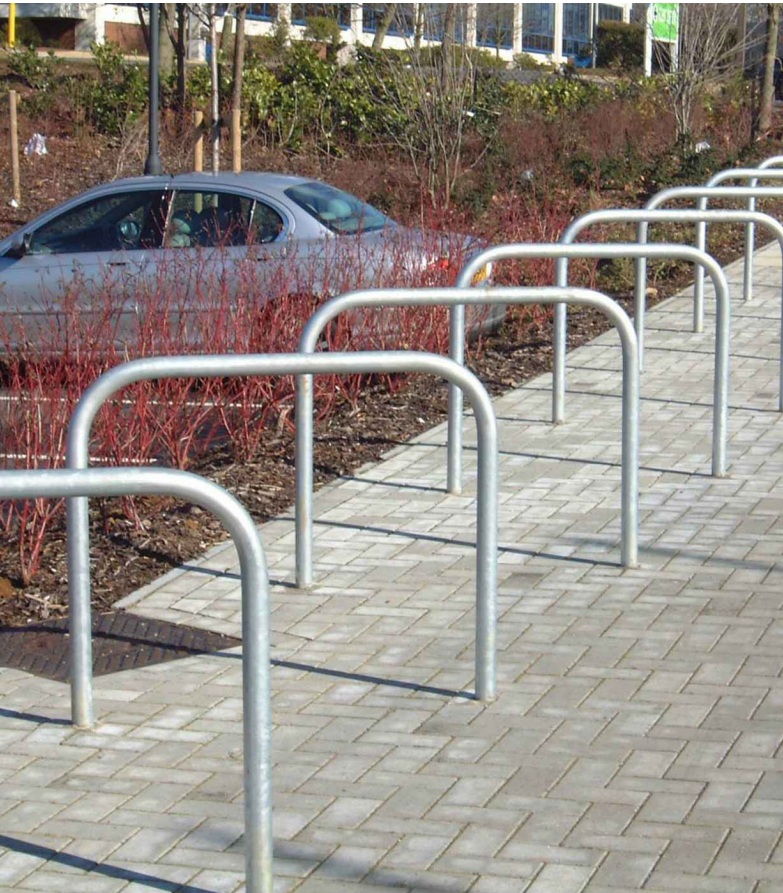
External cycle stands to be Sheffield hoop style of galvanised steel bar construction of at least 3mm thickness
