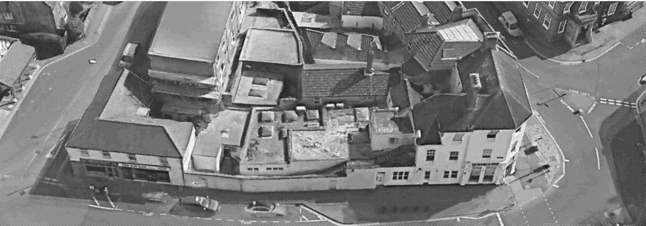
Site and Surroundings
