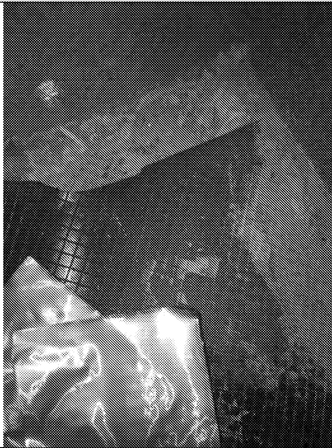
Photograph 25 – Remediated membrane installation
