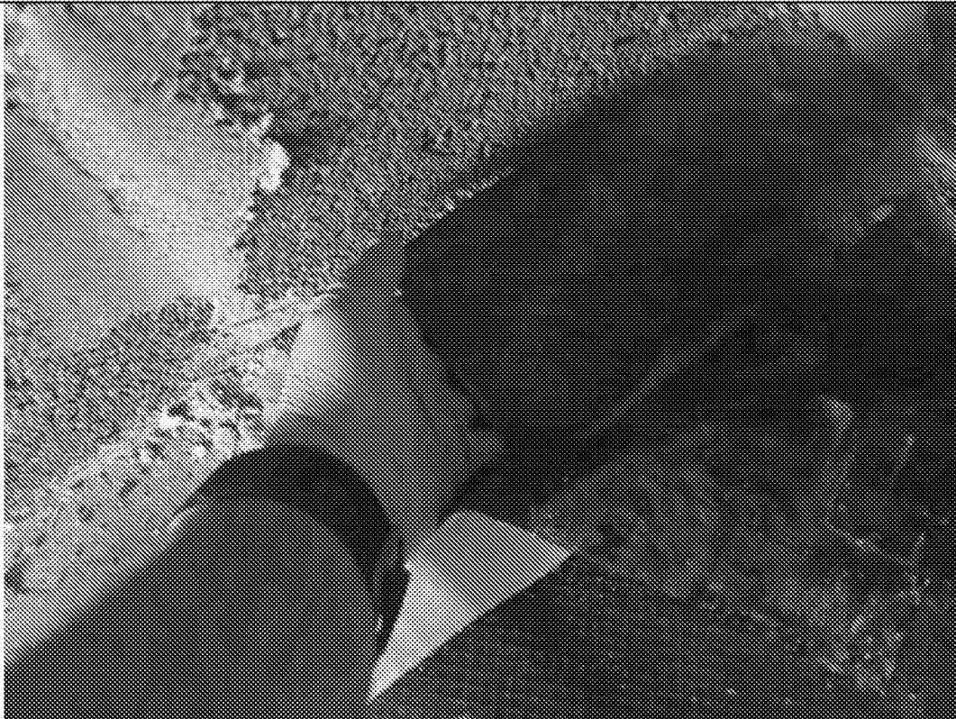
Photograph 33 – Overview of 6-12: Corner Detail not Installed Properly
