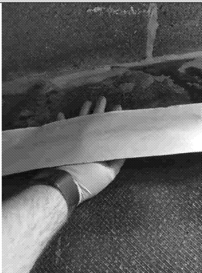
Photograph 29 – Overview of 6-12: Jointing Tape not Installed Properly.
