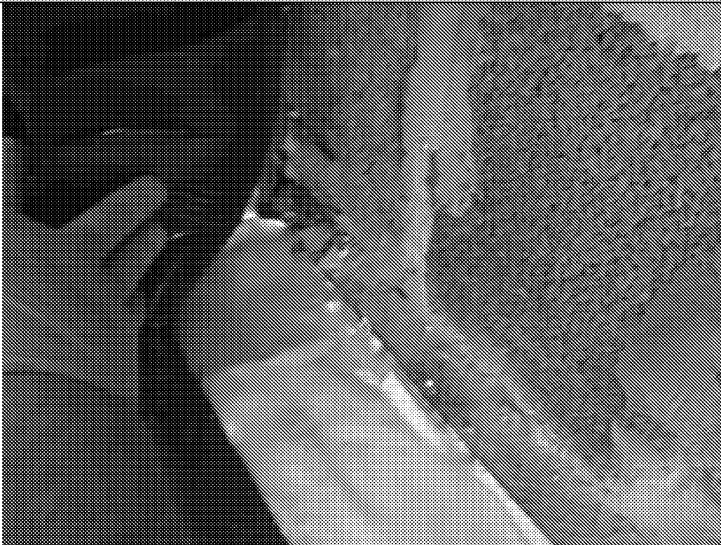
Photograph 37 – Overview of 6-12: Top Hat Detail not Installed Properly
