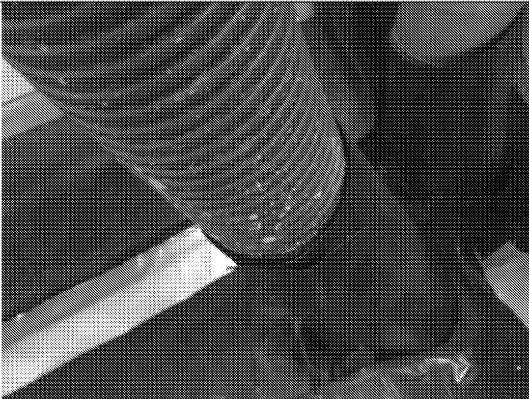
Photograph 37 – Overview of 6-12: Top Hat Detail not Installed Properly
