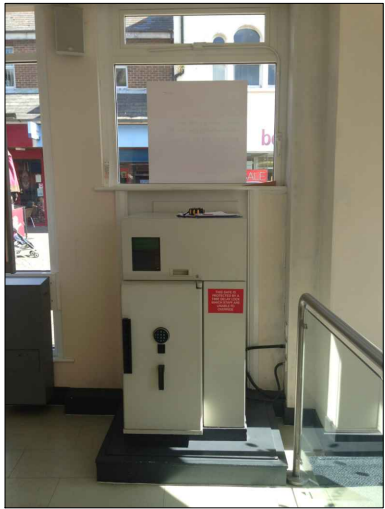
External ATM - Internal View
