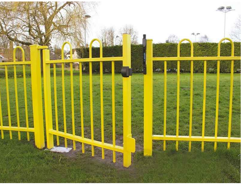
14 Bow top fencing and gates
