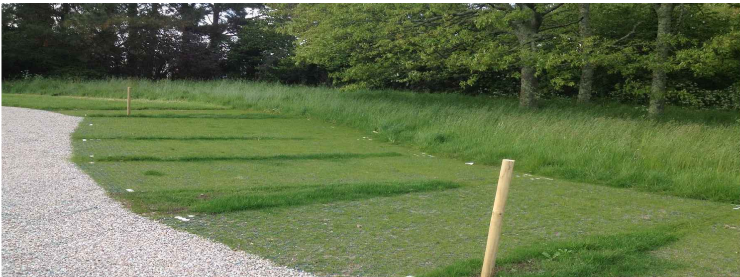
Grass reinforcement - Golpa Grass by Geosynthetics Limited or similar
