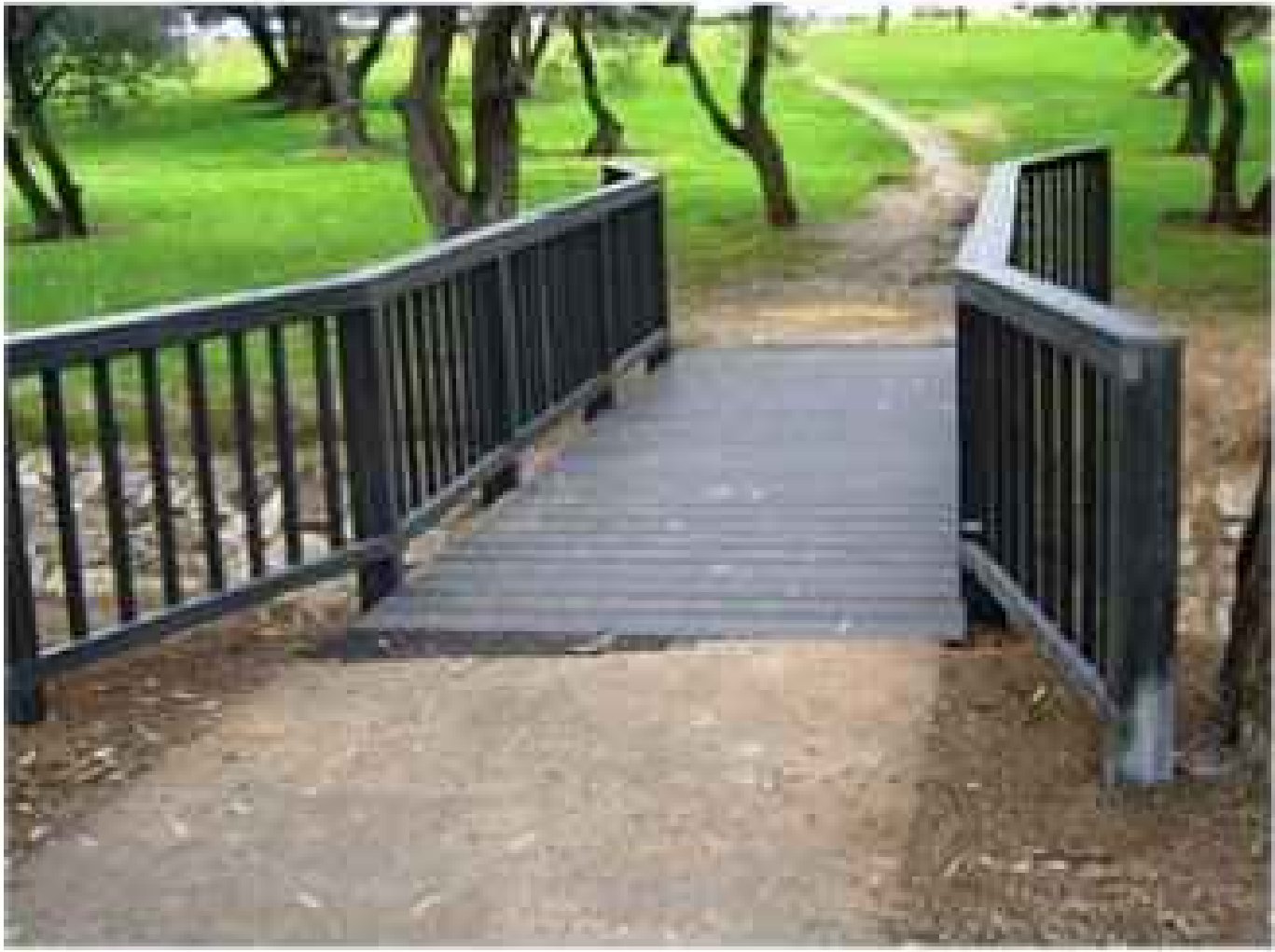
Image above showing example boardwalk over the swales within the CWA. Wood effect plastic.
