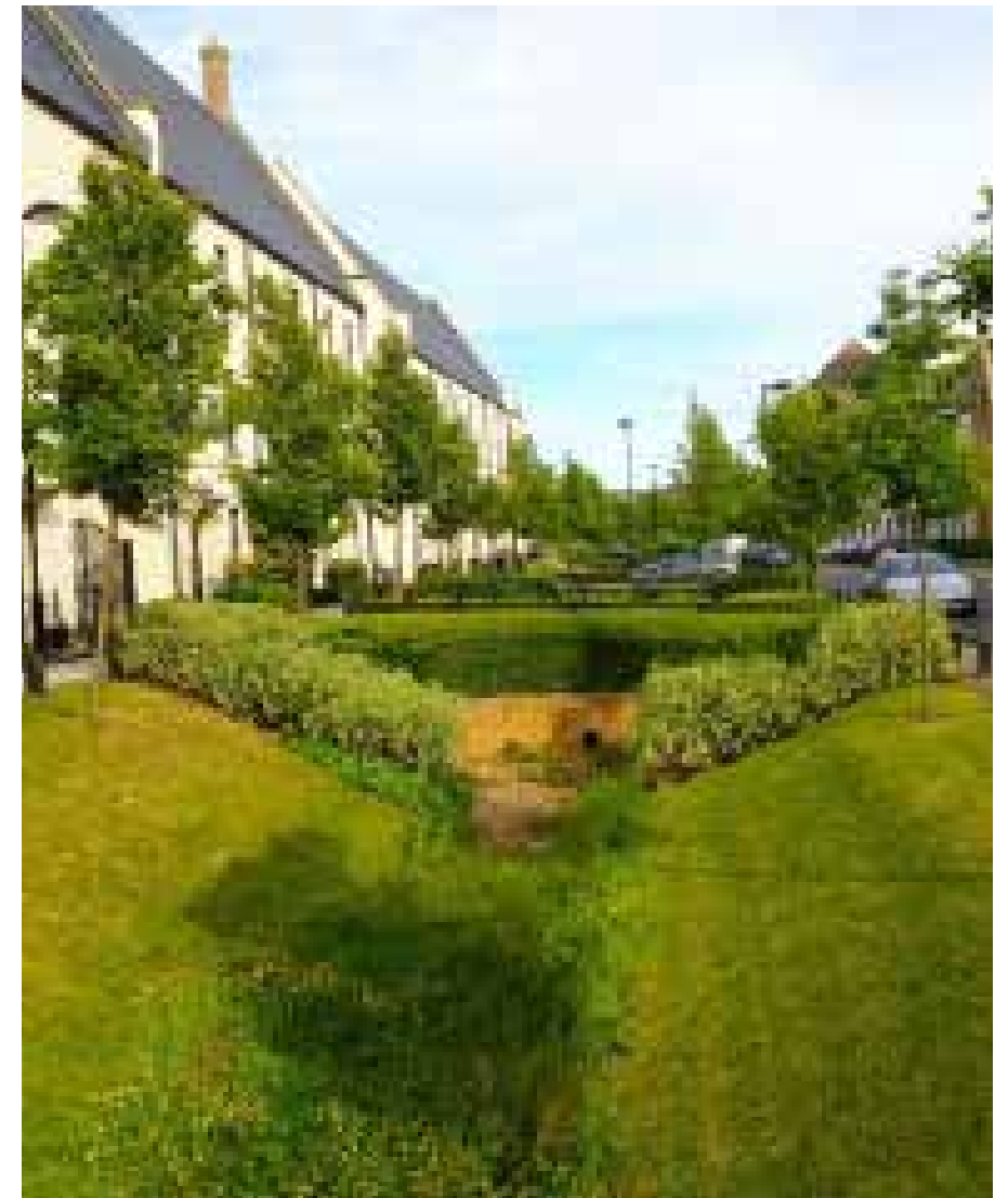
FIGURE 5. ABOVE IS AN EXAMPLE OF THE LINEAR SWALES SIMILAR TO THAT PROPOSED IN PHASE 5. SURFACE WATER WILL BE DIRECTED FROM THESE SWALES TO THE CENTRAL WETLAND AREA; THE LATTER WILL HAVE A DISTINCTLY MORE INFORMAL FEEL IN ITS MEANDERING PATHS AND DRAINAGE CHANNEL'S.
