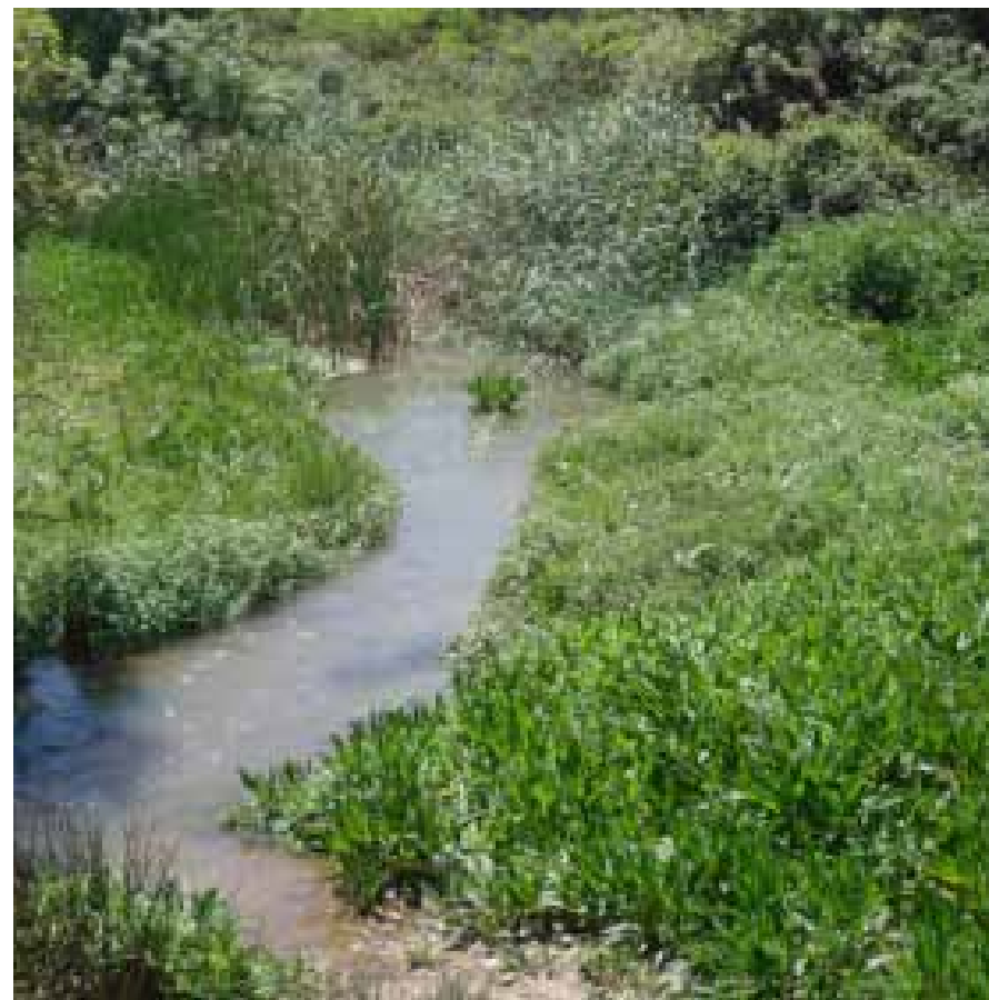
FIGURE 1. THE CREATION OF LOW FLOW DRAINAGE CHANNELS AND WETLAND PLANTING WILL DIRECT SURFACE WATER AND WILL PROVIDE CONSIDERABLE AESTHETIC VALUE TO THE SCHEME. DRAINAGE BASINS LINKED BY A CONTINUOUS SWALE WILL TRAVEL THROUGH THE WETLAND AREA MANAGING THE FLOW OF SURFACE WATER DURING PERIODS OF RAIN, WHILE OFFERING ENHANCED ECOLOGICAL AND HABITAT BENEFIT.
