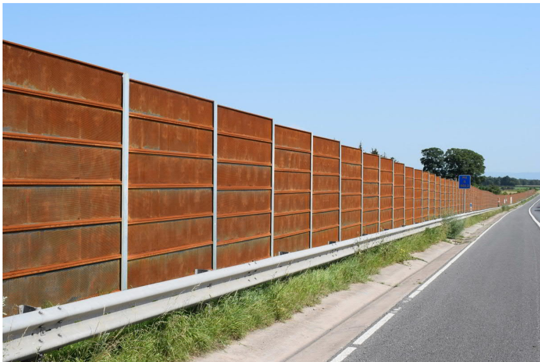
M6 near Carlisle – After steel almost fully weathered
