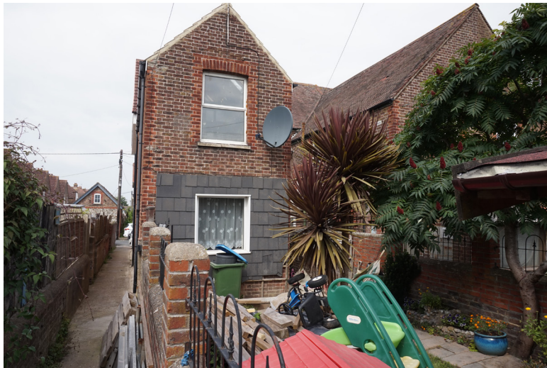
Rear facade incorporating adjoining properties
