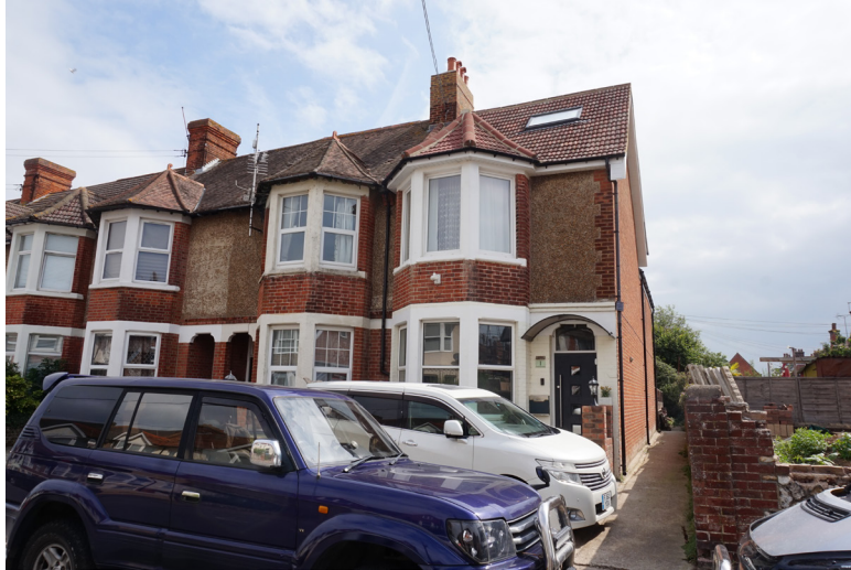
Front facade incorporating adjoining properties
