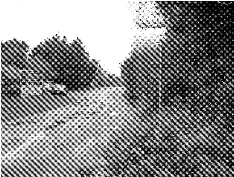
Photo 7 Visibility to the Right (North)
