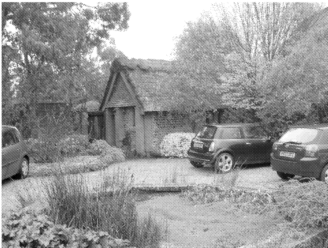
Photo 3 Additional View of Parking in Forecourt
