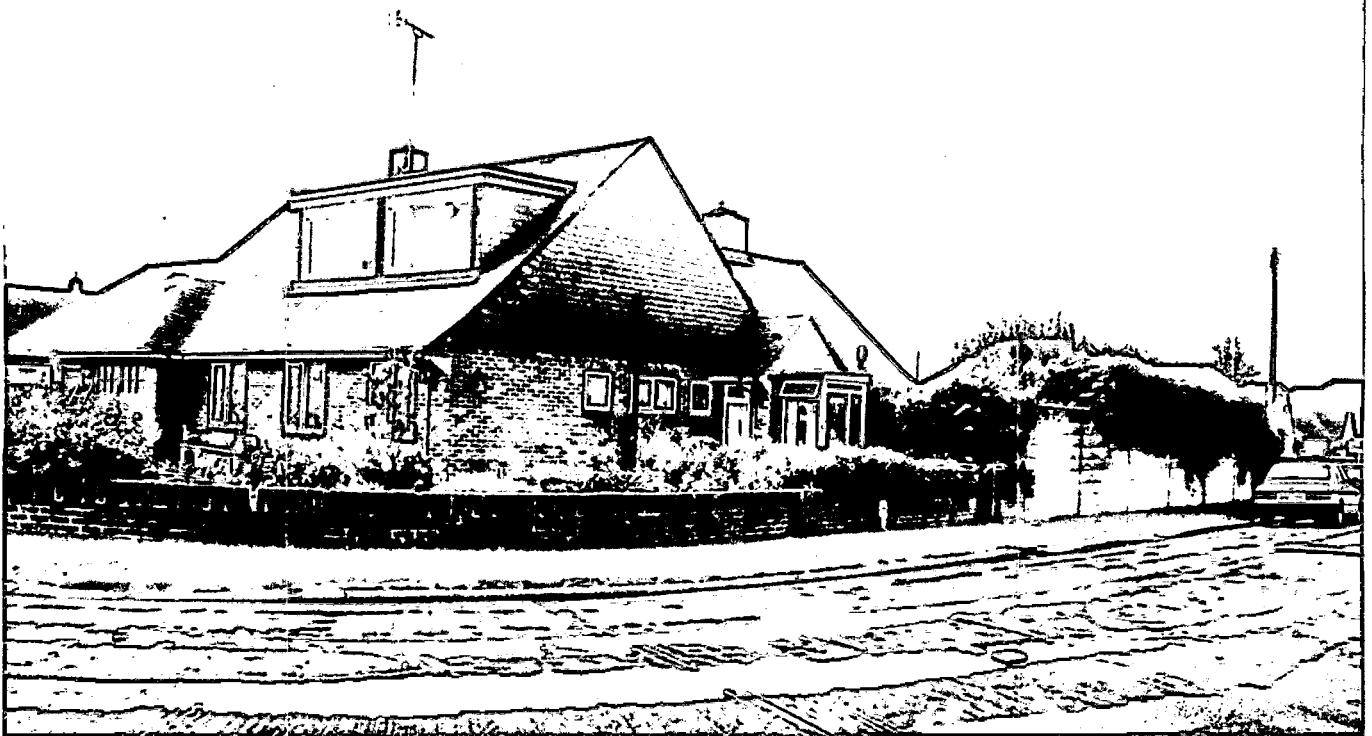
North and East sides of House as Existing
