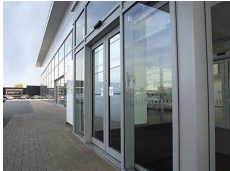
Door: Alluminium frames with 6.4or4-16-4 double glazing Low-E argon filled Colour dark grey
