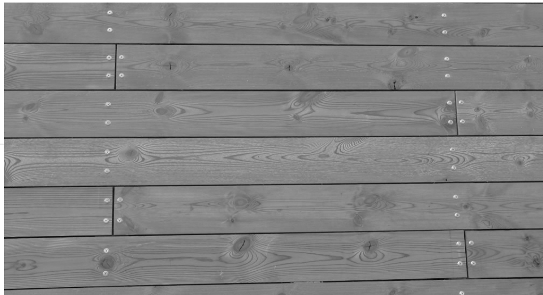
Timber cladding: Thermowood T&G
