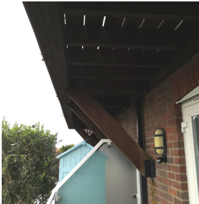
Supports to 32 and 33 Balconies
