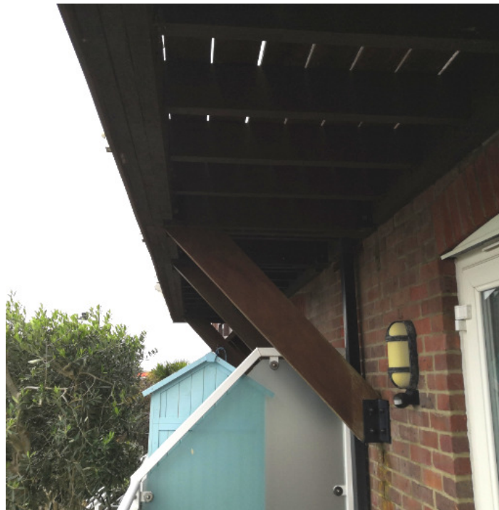
Supports to 32 and 33 Balconies
