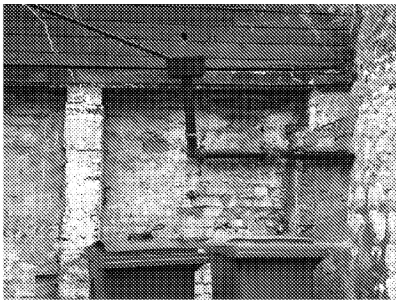
All cement mortar/pointing to be removed
