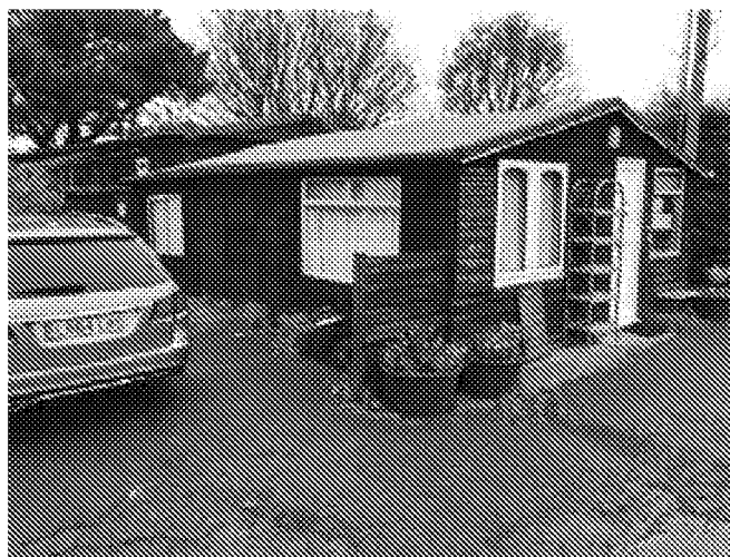
18 Northern Portion Looking North
