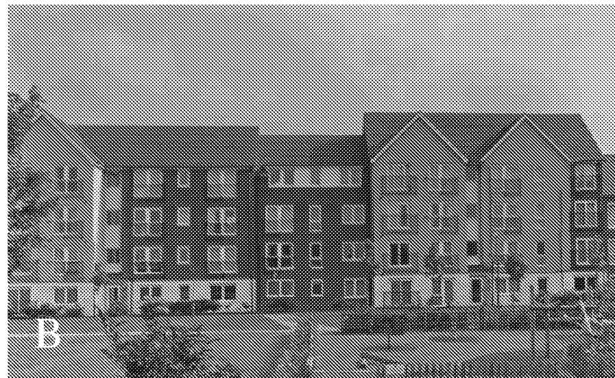
Four storey flats at Gratwicke Drive (site to north of A259)
