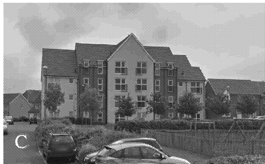
Combination of three and four storey flats and two storey houses at Stammer Road (site to north of A259)
